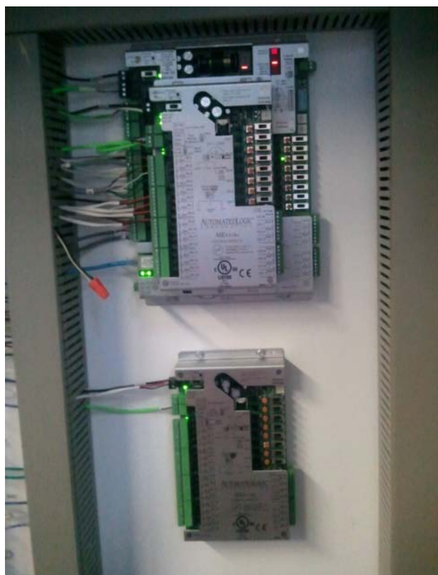
Figure 33 – The ALC data acquisition boards for analog and MODBUS signals.
