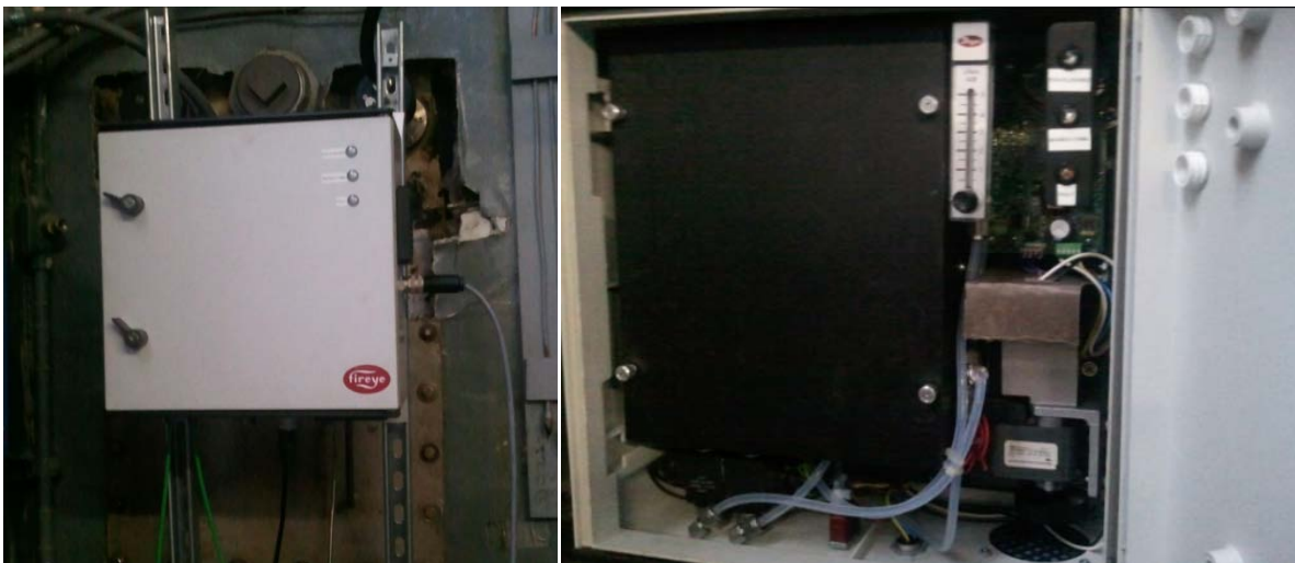
Figure 17 – The Fireye box, used for CO and O 2 monitoring and closed loop control.
