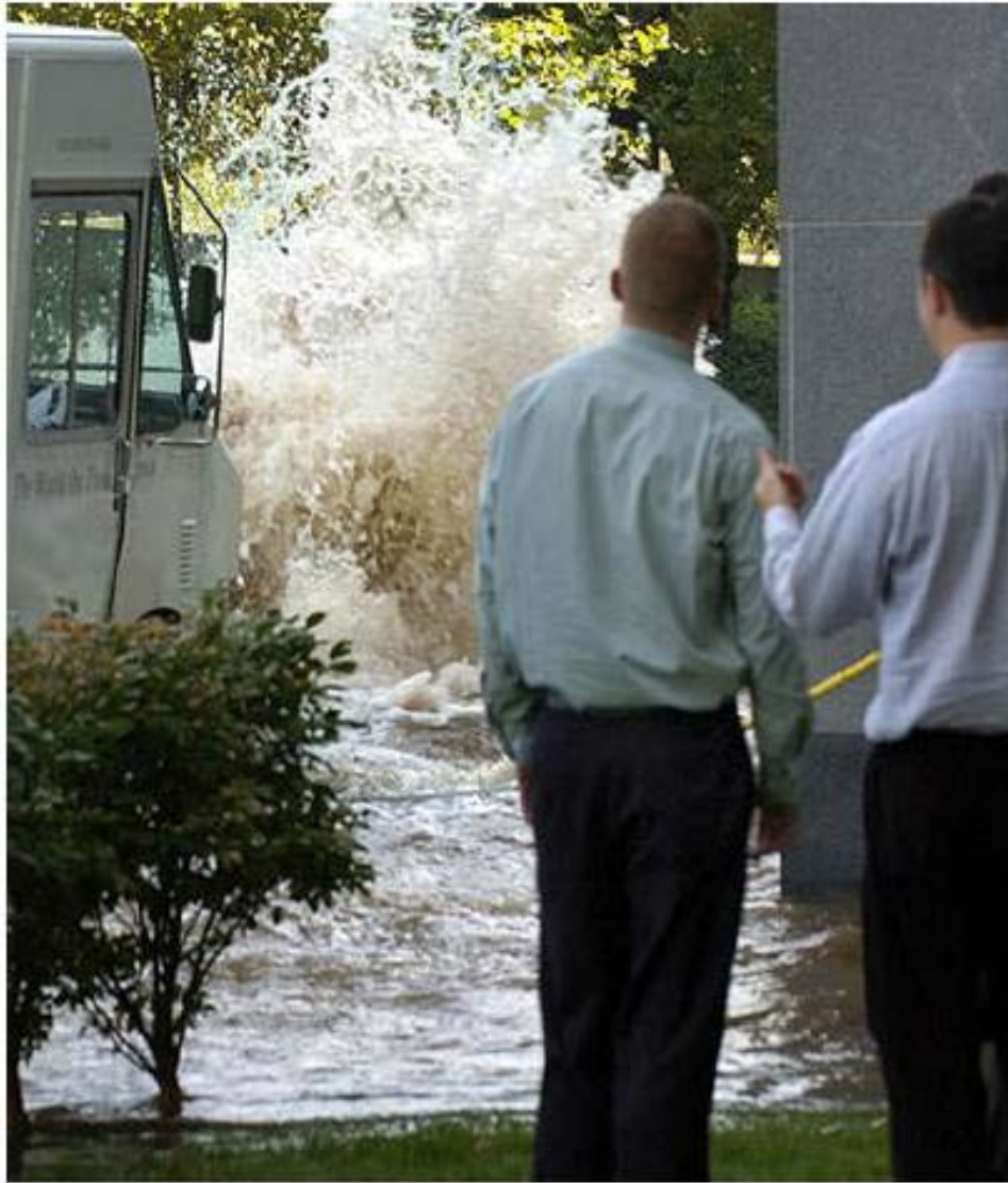
36 Inch Main Break
