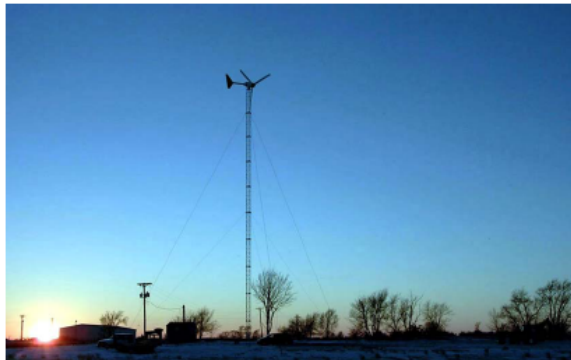
Groundwater recirculation well powered by a wind turbine at the Former Nebraska Ordnance Plant Superfund Site, Mead, NE. Photo by Ernie Gutierrez and used with permission of Curt Elmore, Missouri University of Science and Technology
