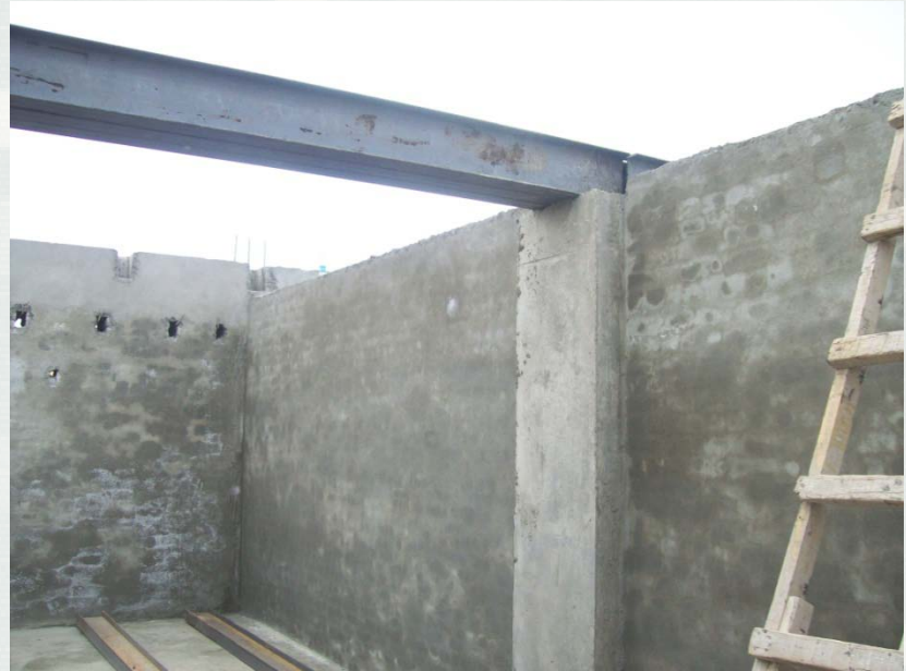
Installing roof beams
