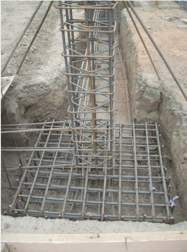
Concrete column prep
