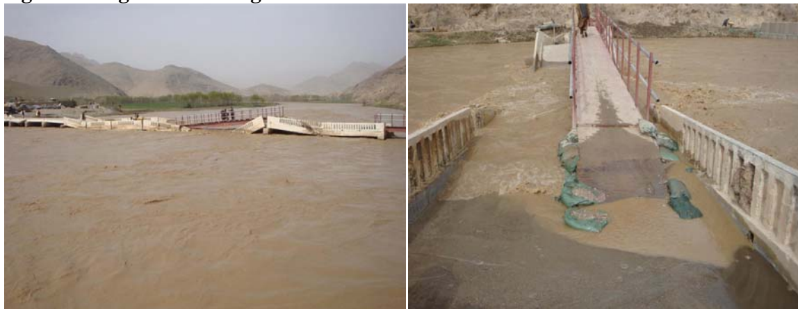
Figure 2. Regak Foot Bridge
