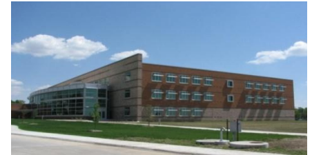
AF Weather Agency – 1 st LEED Gold
