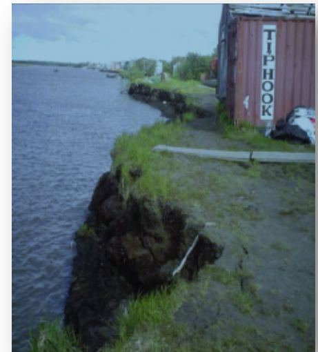
Bank erosion along the Kotlik shoreline, 2007
