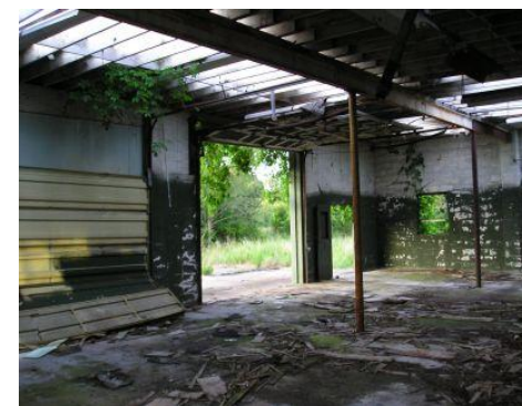
Abandoned buildings at Camp Crowder
