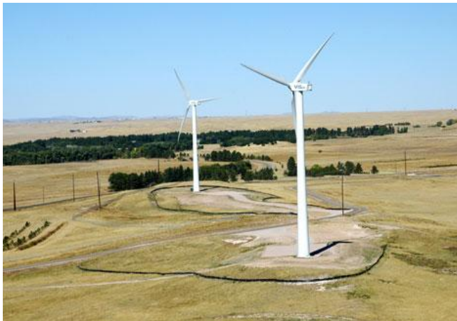
Wind Turbines at F.E. Warren AFB, WY
