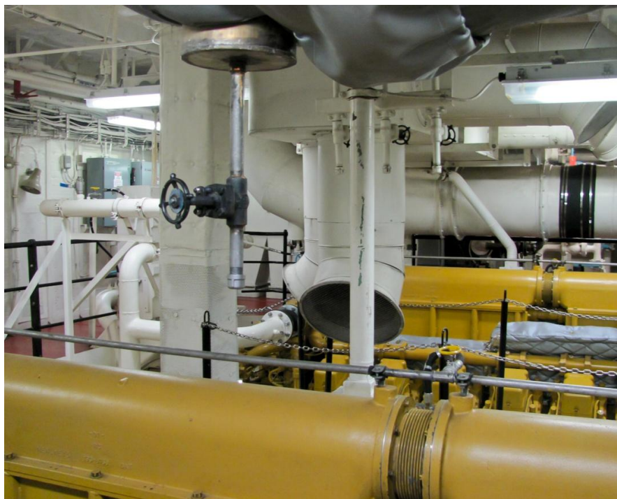
Figure 10. Engine Room Upper Deck (average illuminance 465 lx).
