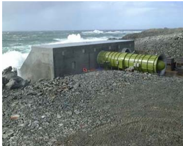
Figure 5. Onshore LIMPET Wave Energy Converter. From [3]
