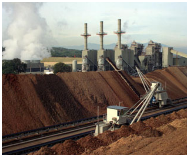
Figure 10. Biomass Power Plant
