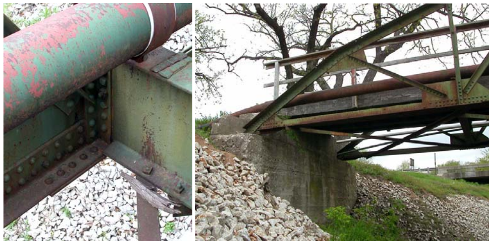
Figure 18. Deck beam-truss connection (left) and cross-bracing (right), (ERDC-CERL 2009).
