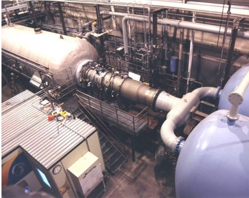
Figure A.18 - Image of the AFRL Turbine Research Facility (TRF).
