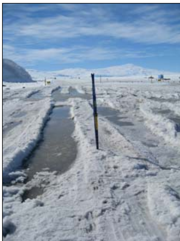
Figure 7. Melted condition of Scott Base Transition on 20 January 2008.
