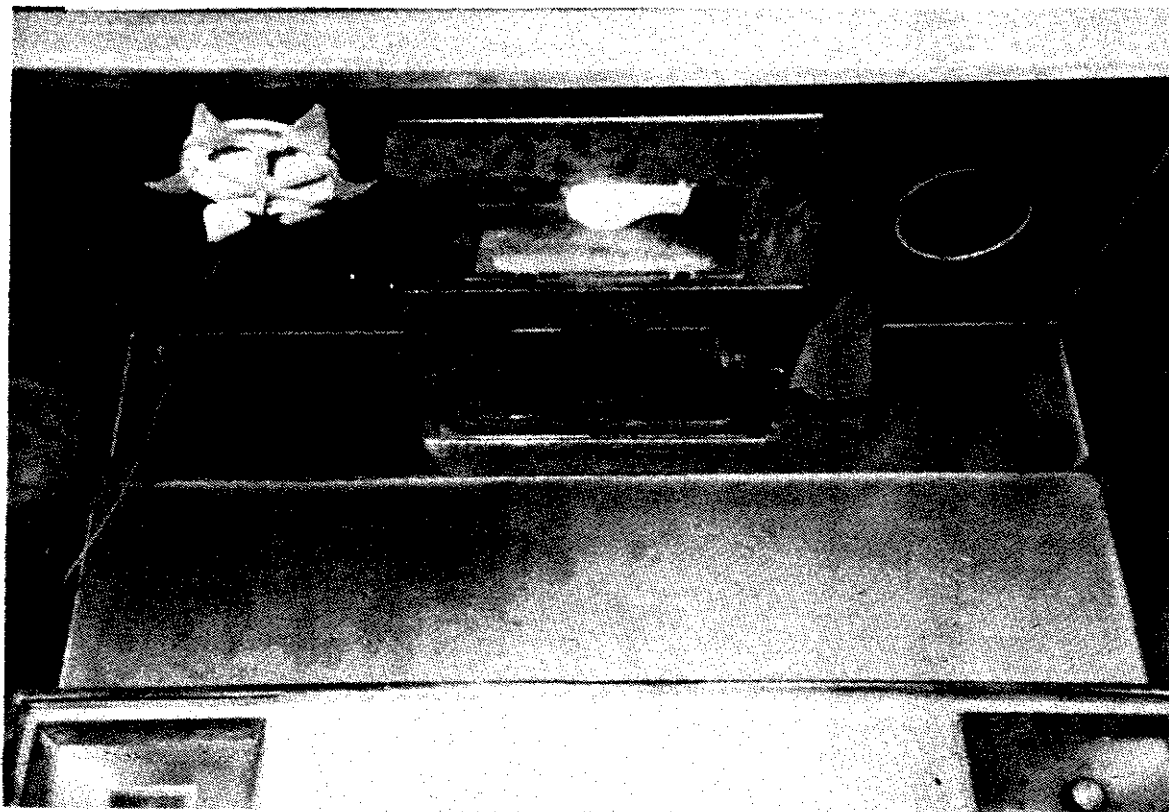
Figure 1. Range Queen Kitchen Range Fire-Extinguishing Device
