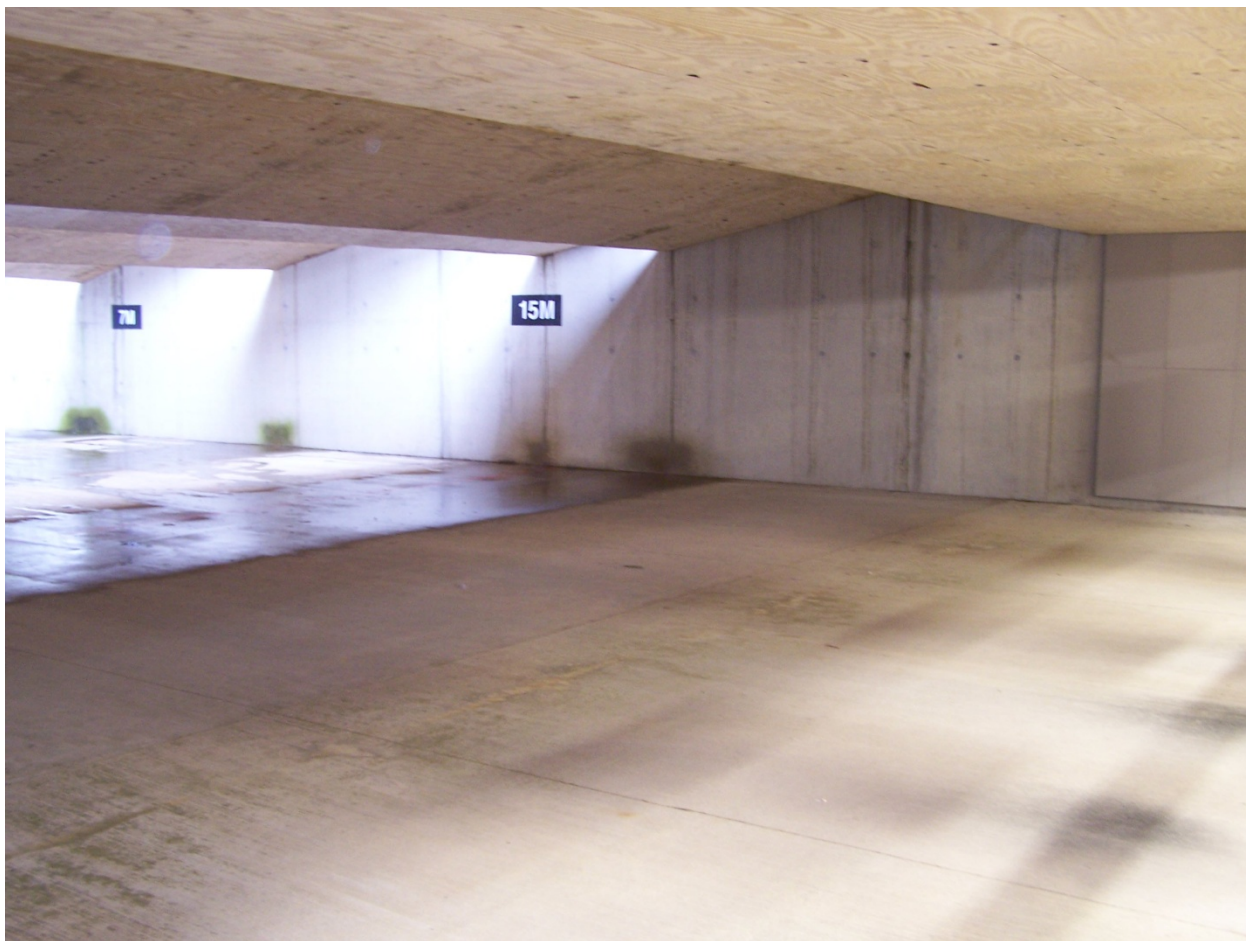
Figure 3. Side wall and overhead containment baffles
