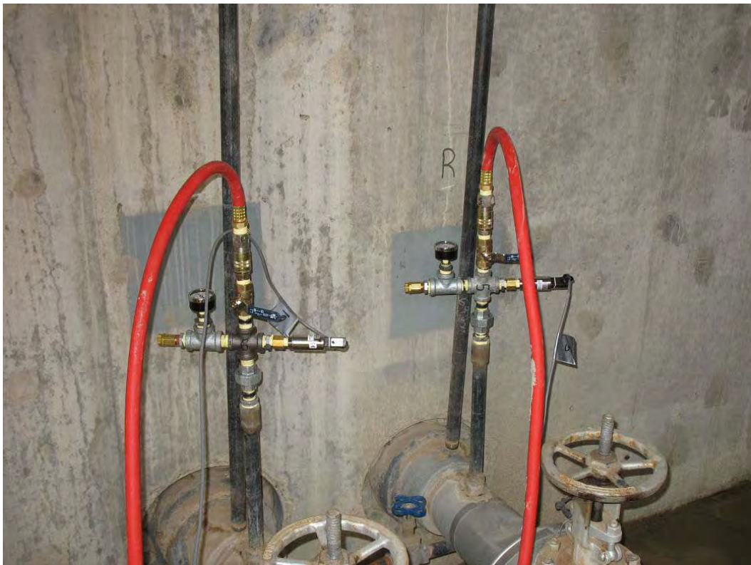
Figure C4. Conduit pressurization test rigs.
