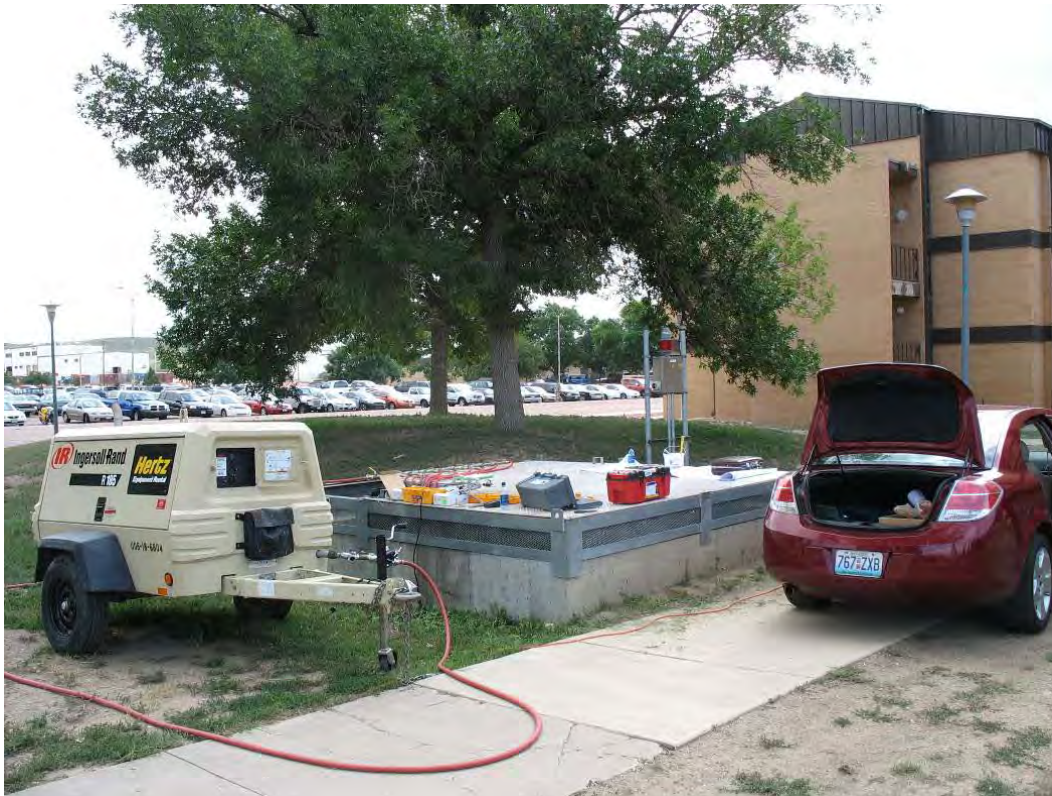
Figure C1. Pressure check field setup at Fort Carson.
