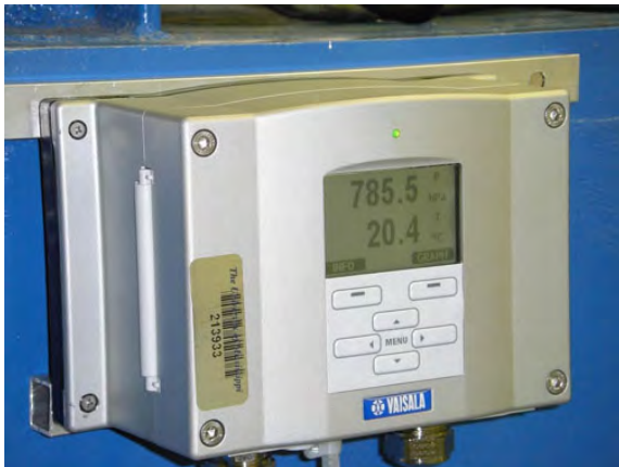
Figure 7: The Vaisala pressure and temperature display unit is shown mounted on the chamber side wall.
