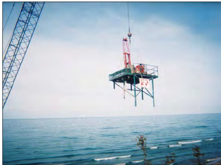
Figure 34. Green drilling platform and red drill at MPS suspended by 100-ft crane. Stairs have been rebuilt three times by property owners because of slope failures (photos after STS 2005).
