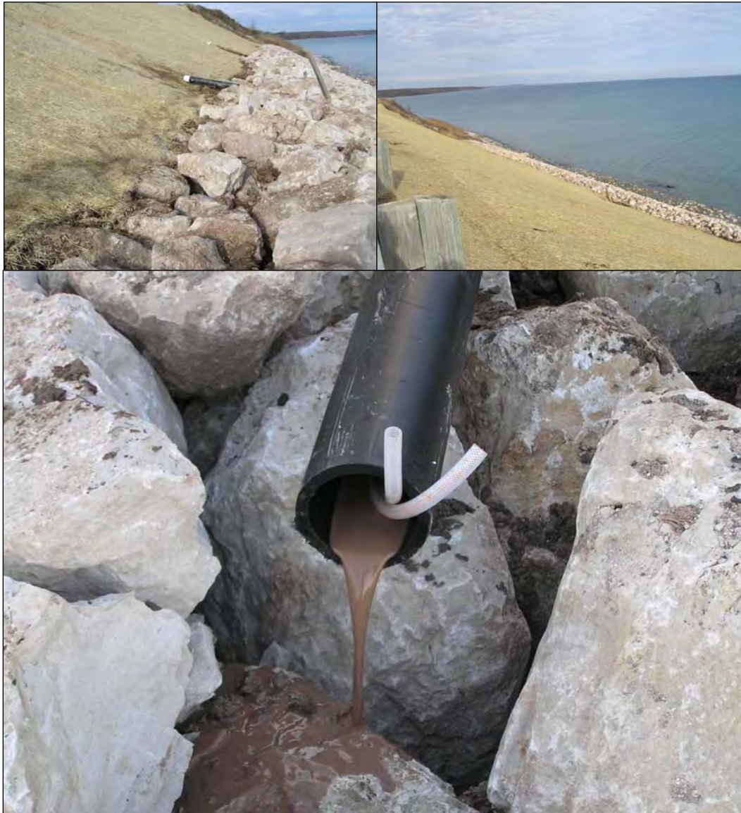
Figure 52. Slope, clockwise from top left, after cut and fill of the surface material; installation of gravity drains and toe revetment; and view of drain outlet at the revetment just after construction (photos courtesy of Ross, USACE, Detroit District).
