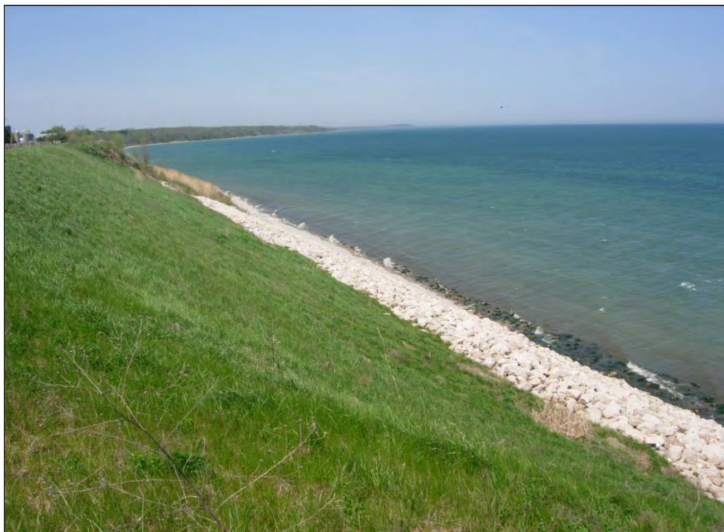
Figure 53. View after construction of gravity drained Mosel Bluff, Sheboygan County, Wisconsin. Note heavily constructed revetment at toe to prevent foreshore erosion (photos courtesy of Ross, USACE, Detroit District).
