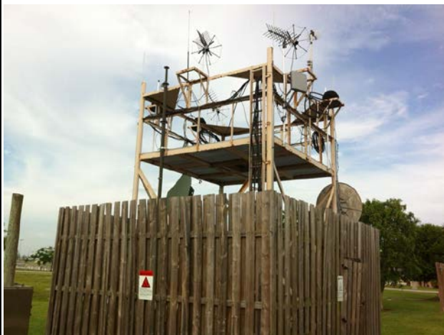
Figure 1: Special Operations Command South Antenna Cluster
