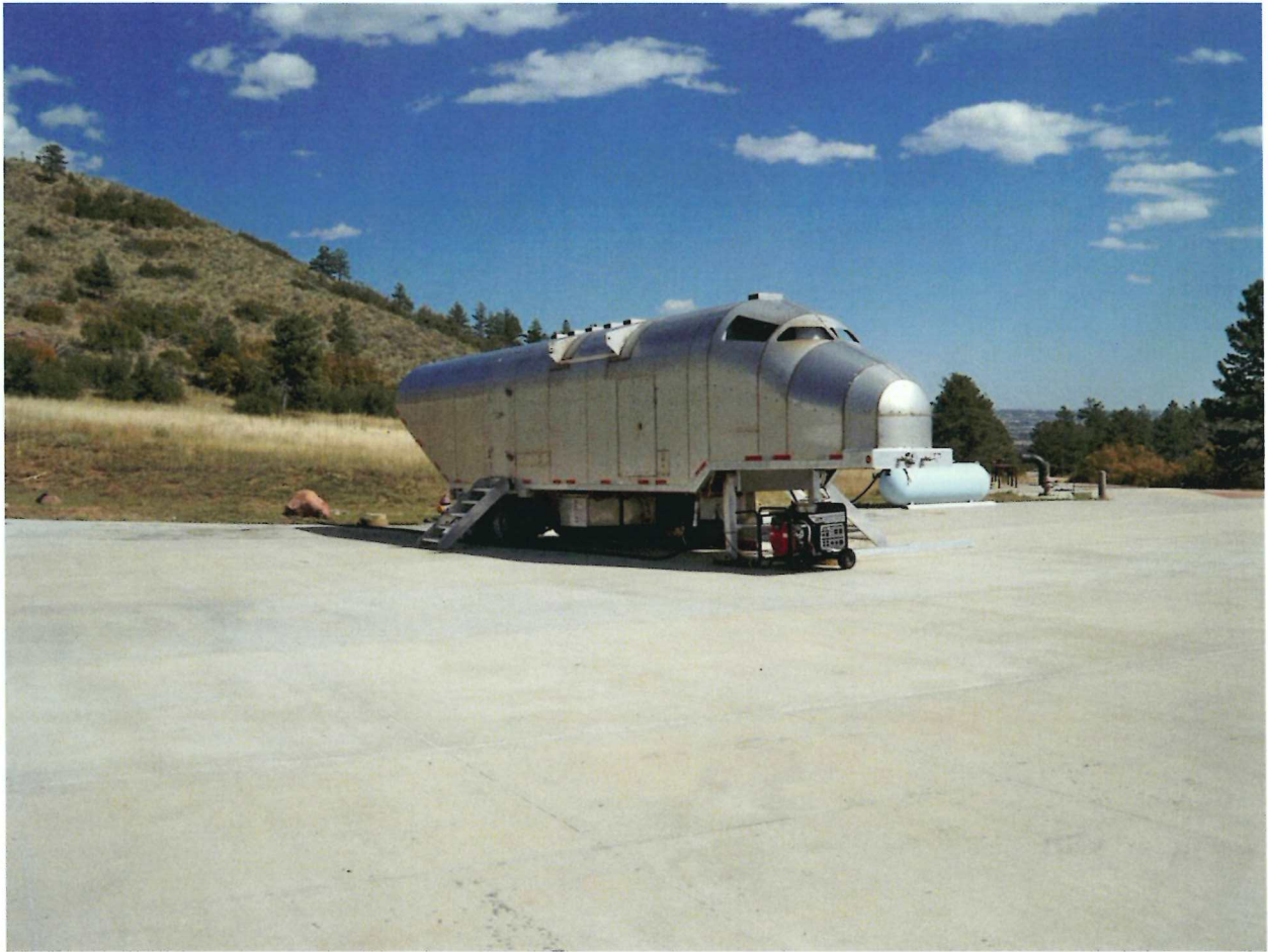
Photograph #2, The Existing MAFT Looking Northeast From Access Road.
