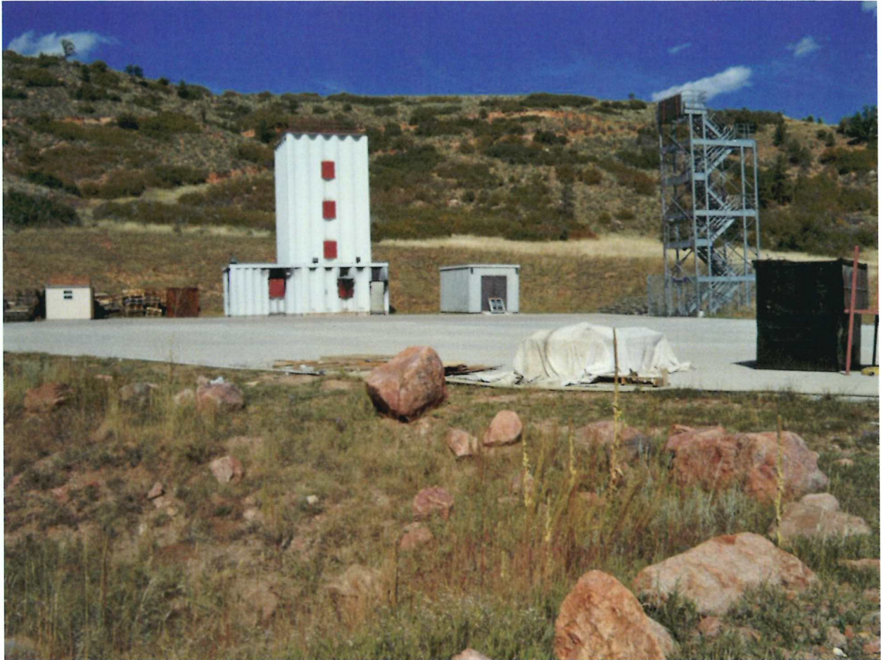
Photograph #1, Existing MAFT Looking North From Access Road.
