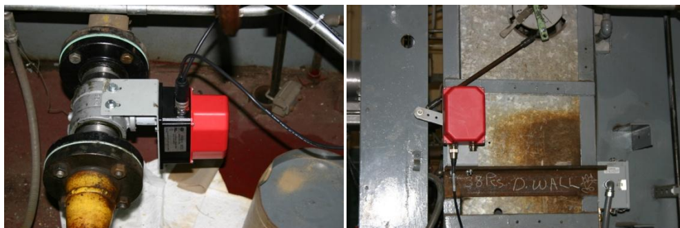
Figure 7. Fuel/air positioning electromechanical actuators. Fuel servomotor on left, air servomotor on right.
