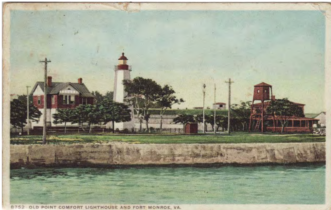
Figure 166. Post card of lighthouse, keeper's house and fog bell, date unknown (Casemate Museum).
