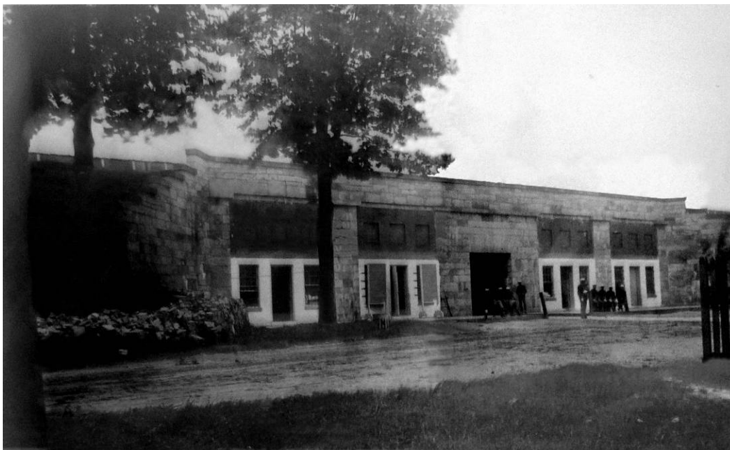
Figure 87. Guard house at main gate, date unknown (Casemate Museum).
