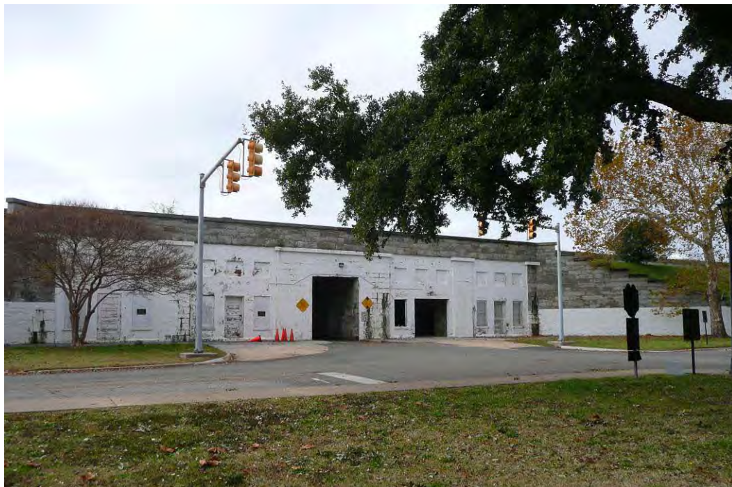
Figure 89. Guard house at main gate, 2009.
