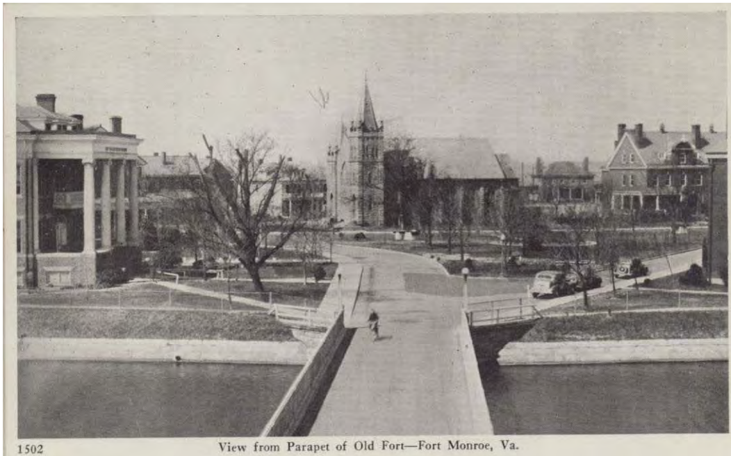
Figure 137. Looking west from Main Gate, 1920 (Casemate Museum).
