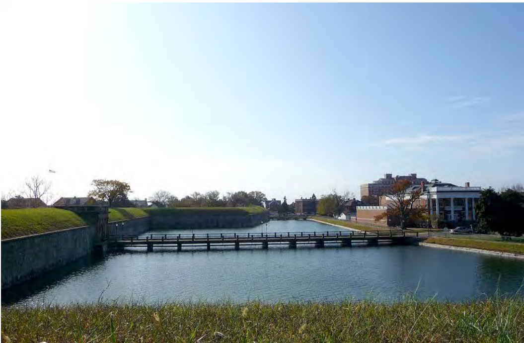
Figure 141. View south towards Main Gate, 2009.
