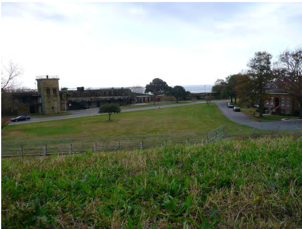
Figure 183. View from third front, 2009.
