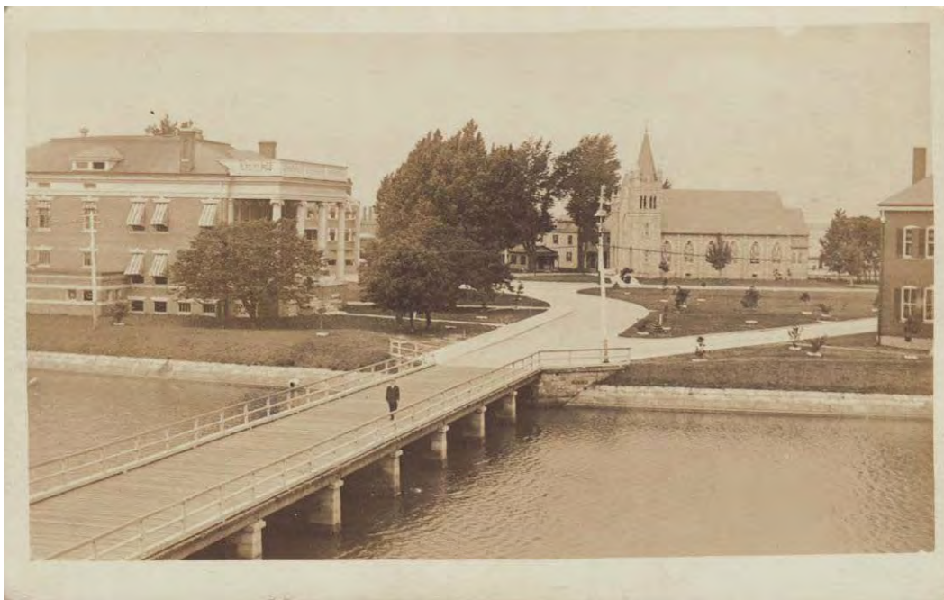
Figure 136. Looking west from Main Gate, 1920 (Casemate Museum).
