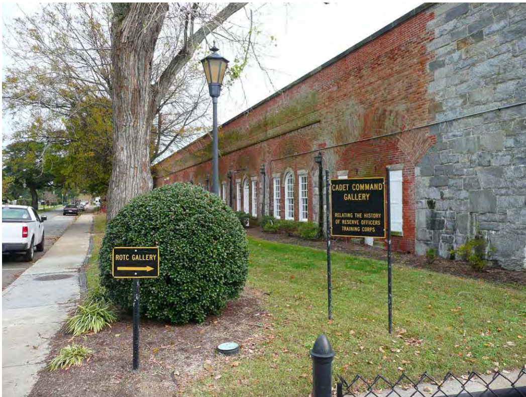
Figure 79. Casemates of the second front, 2009.
