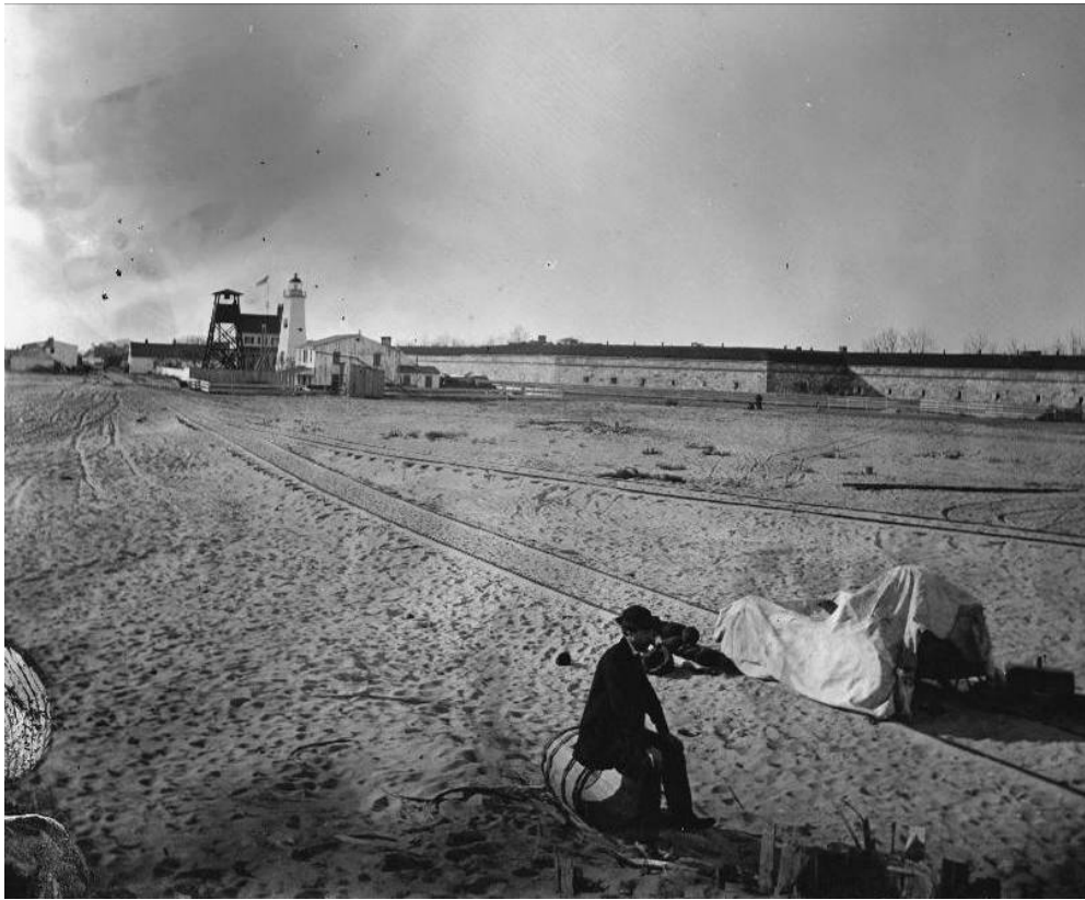
Figure 4. Point Comfort Lighthouse in 1864 (Library of Congress).
