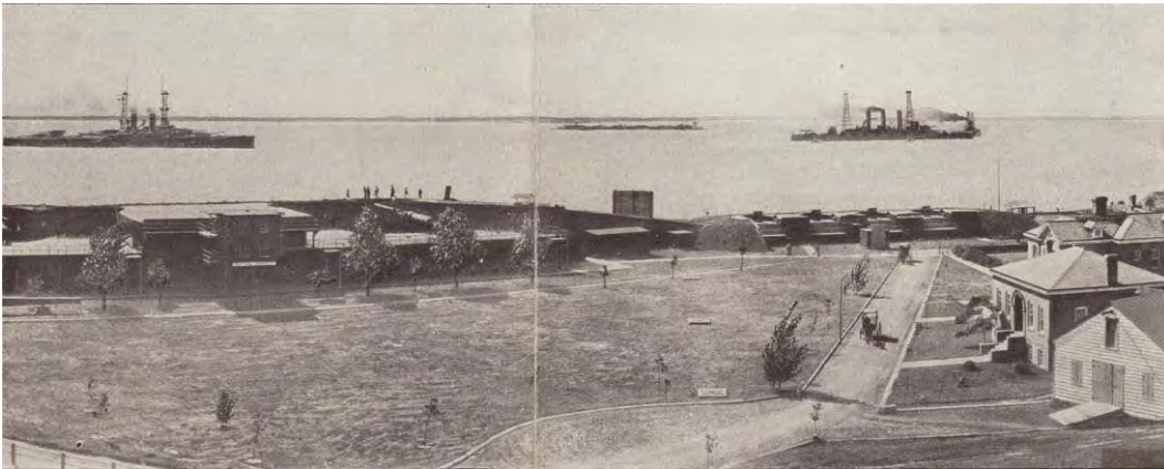
Figure 182. View of Batteries Parrot and Irwin from the Fort, date unknown (Casemate Museum).
