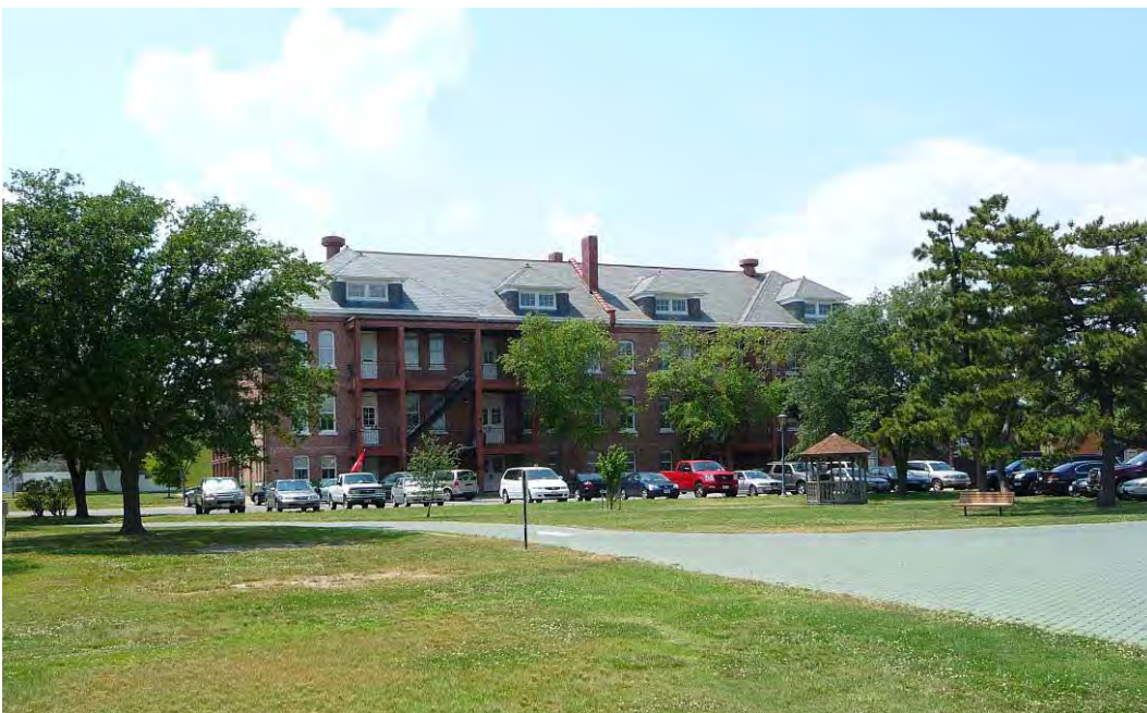
Figure 56. View toward Building 10, 2009.
