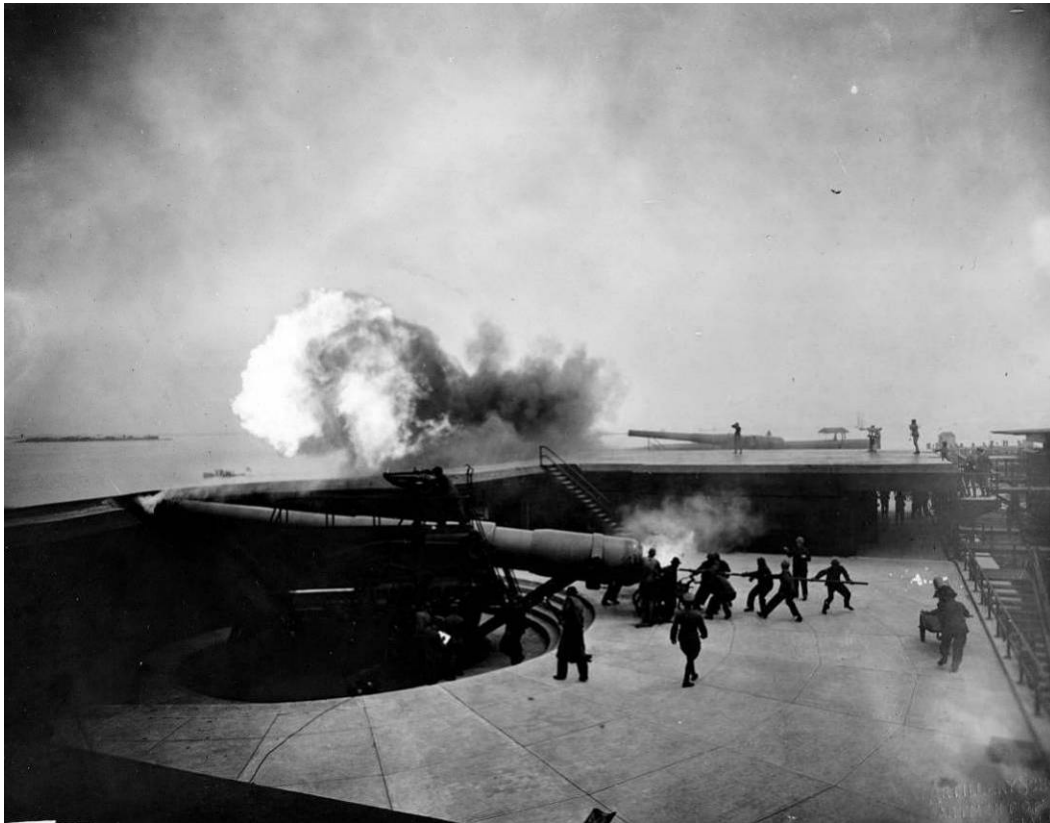
Figure 21. Batteries, 1918 (NARA College Park).
