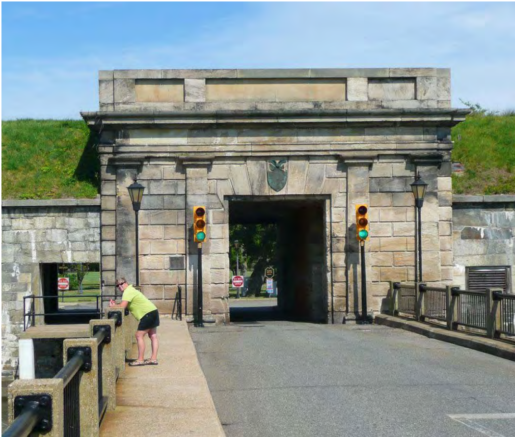
Figure 146. View of Main gate, 2009.
