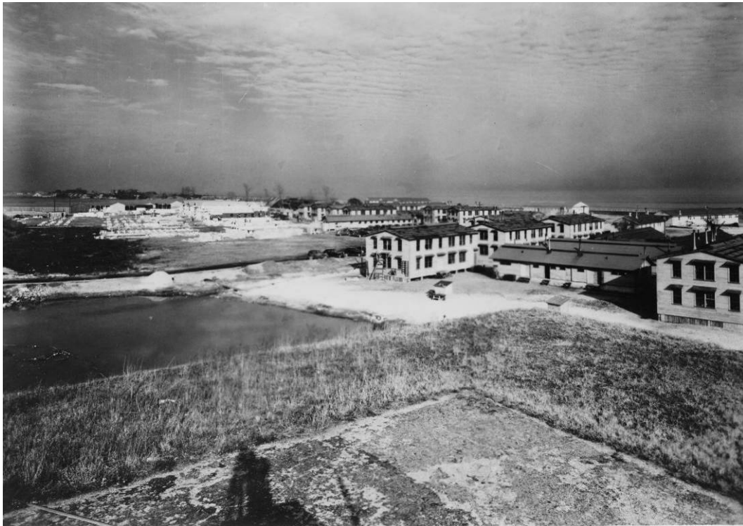
Figure 186. View from the fifth front (Fort Monroe Cultural Resources).
