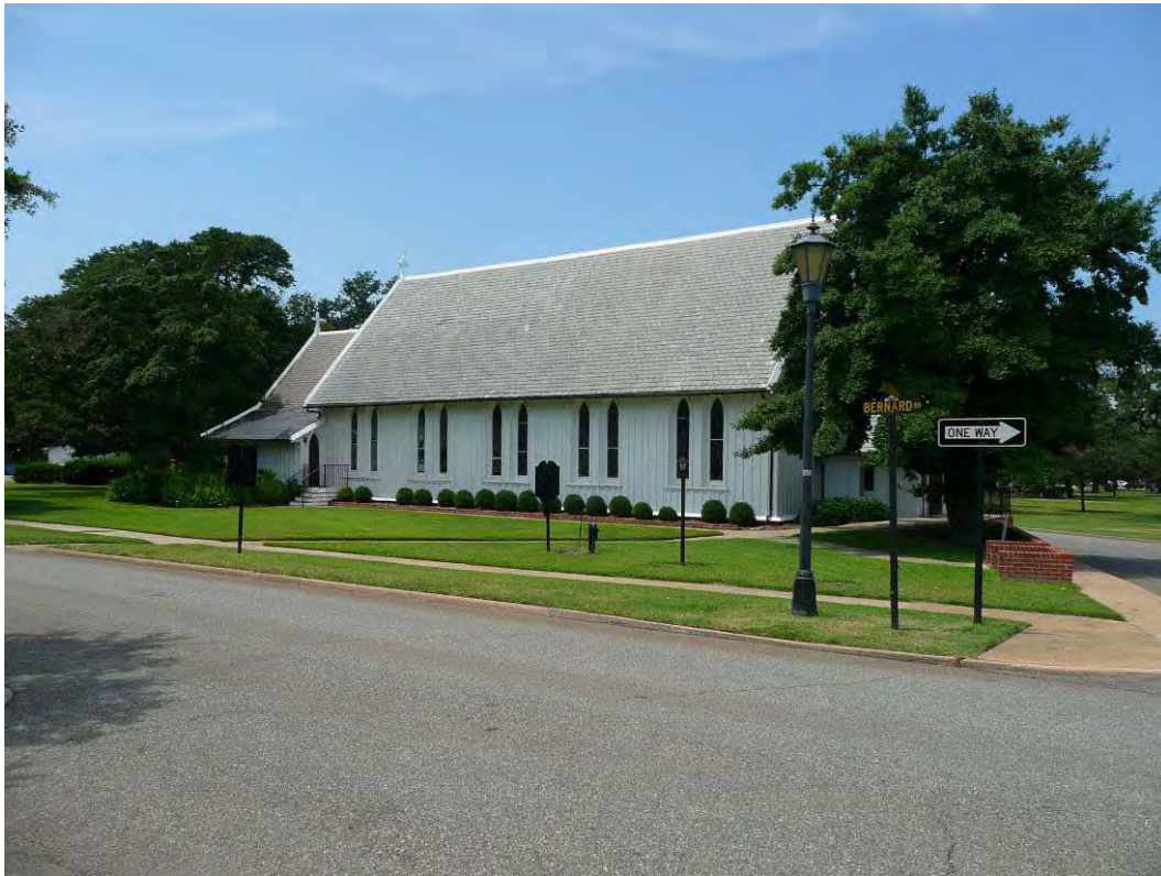
Figure 61. View north toward chapel, 2009.
