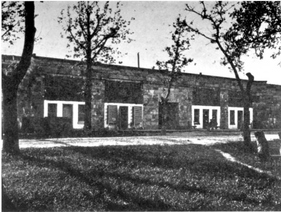
GUARD HOUSE AND MAIN GATE From the interior of the fort about 1890
