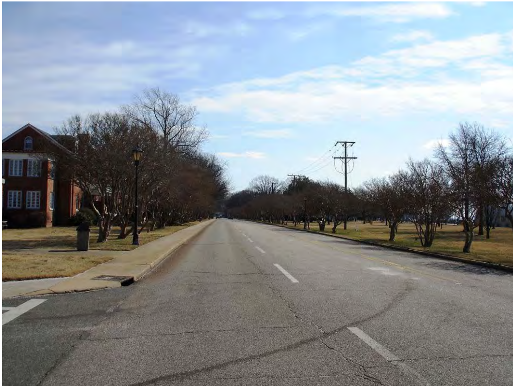
Figure 194. View down Ingalls Road from entrance, 2010 (Fort Monroe Cultural Resources).
