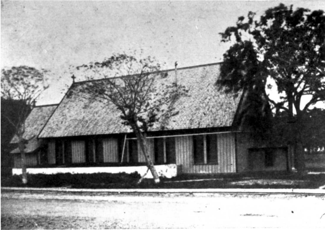
THE POST CHAPEL ABOUT 1885 Note the cistern beside the chapel
