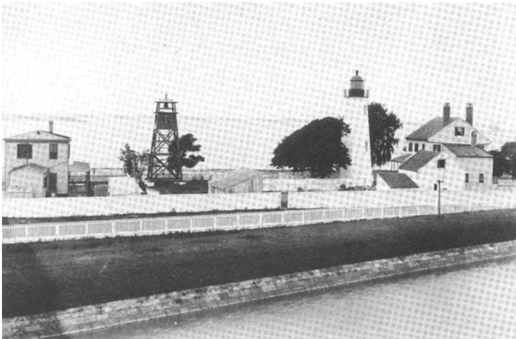
Figure 160. View towards Fort Wool, 1885 (Fort Monroe Cultural Resources).
