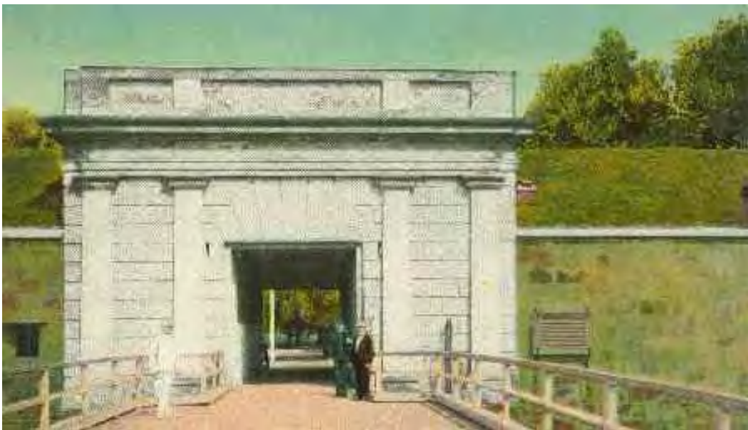
Figure 143. Post card of Main gate, date unknown (Casemate Museum).
