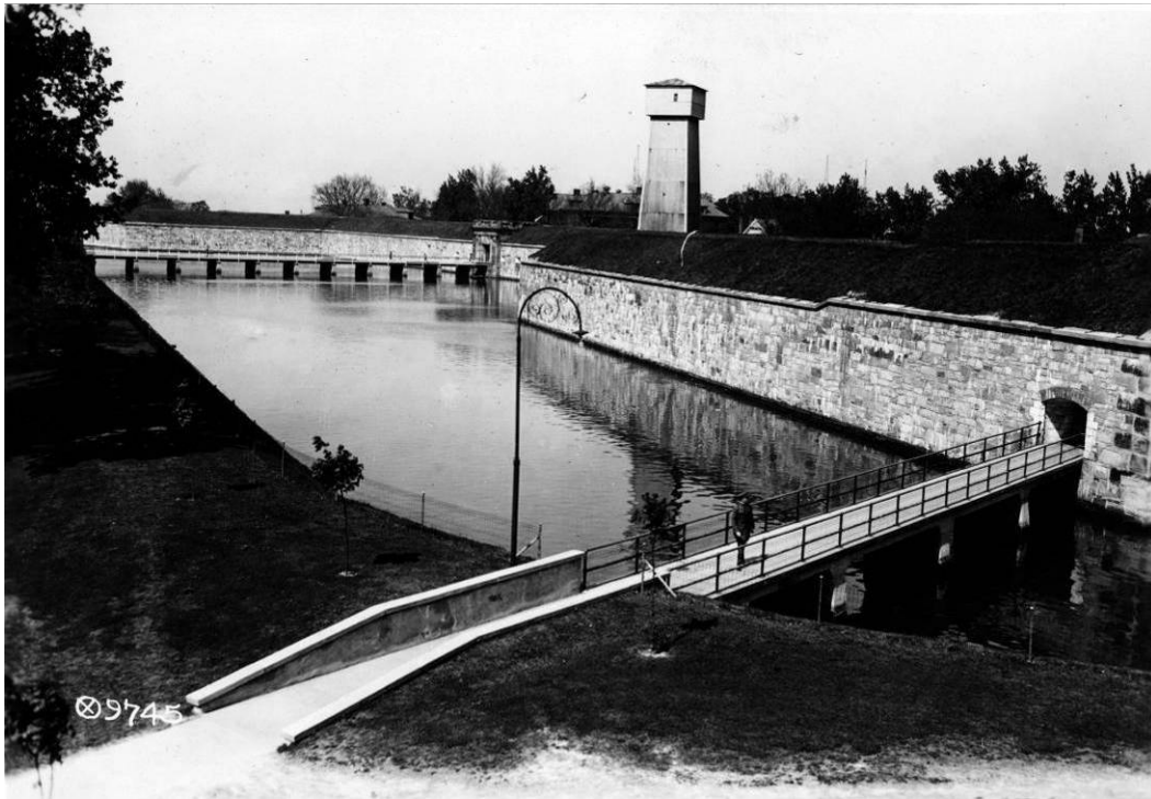
Figure 112. Looking at the postern gate, 1918 (NARA College Park).
