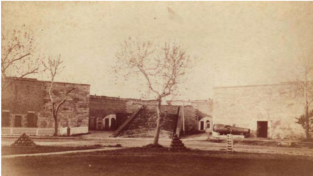
Figure 65. Interior of flagstaff bastion, 1884 (Casemate Museum).
