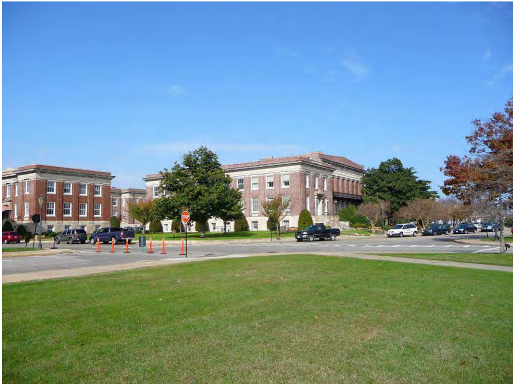
Figure 129. Former Coast Artillery School buildings, 2009.
