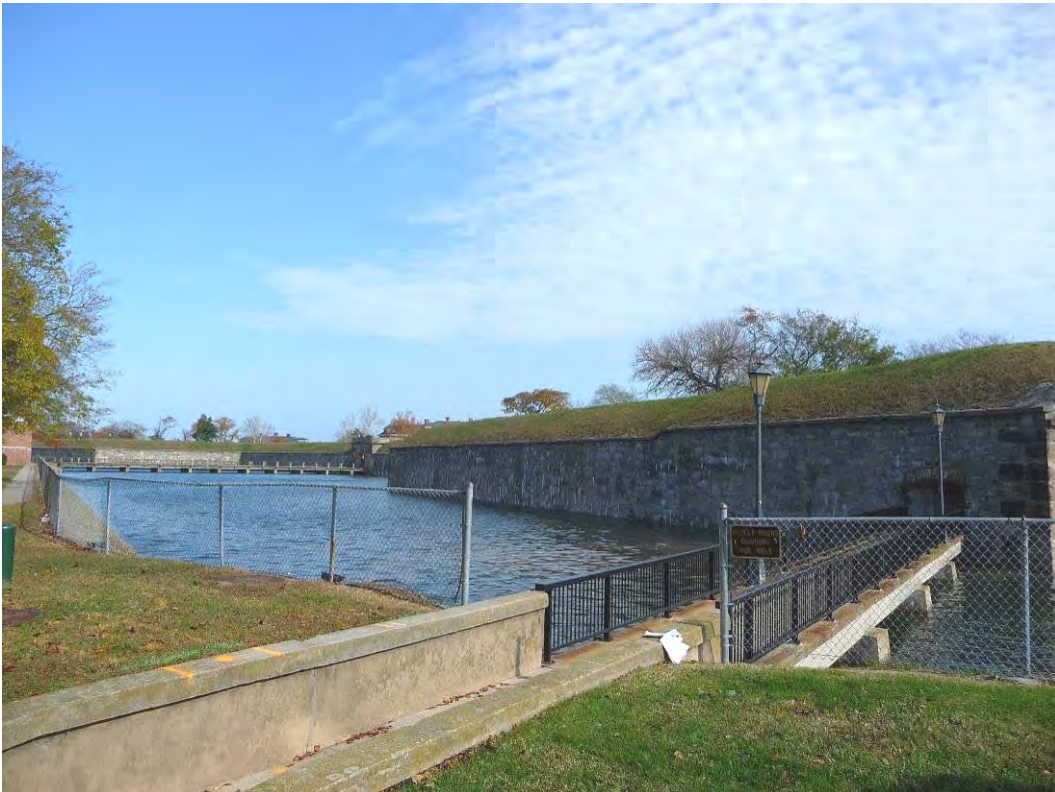
Figure 113. Looking at the postern gate, 2009.
