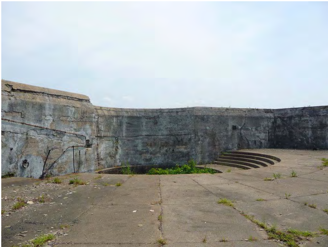
Figure 175. View of Battery DeRussy, 2009.
