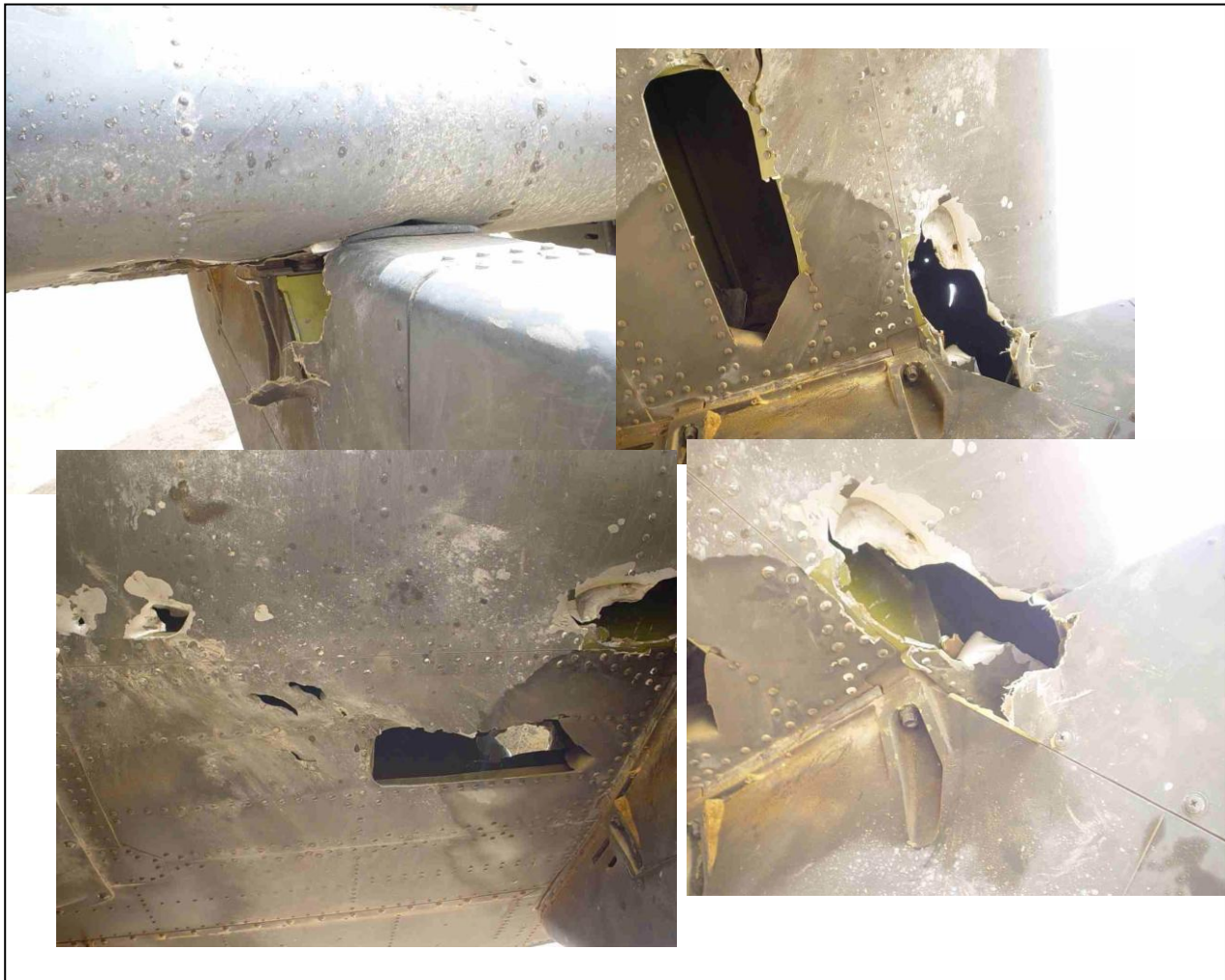
Figure 3: Apache Battle Damage Example, Close Up
