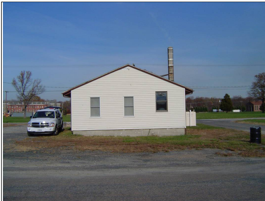
Figure 3-40. APG Building 4031: View of the South Exterior (to the right is E)
