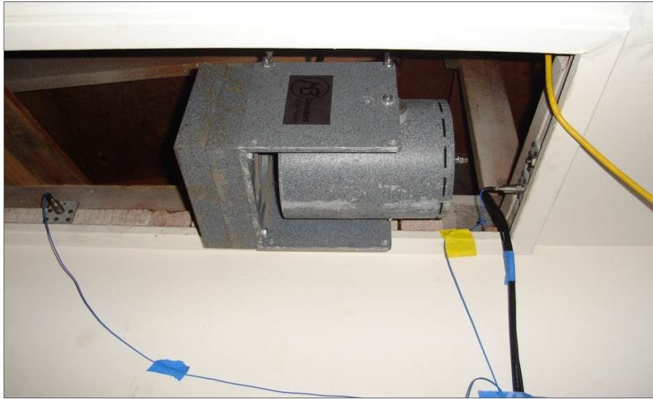
Figure 3-64. Fort Sill, Building 1230: Shaker Installation for Modal Test
