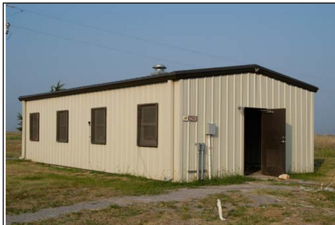
Figure 3-47. Building 6429 at MK19, Fort Sill
