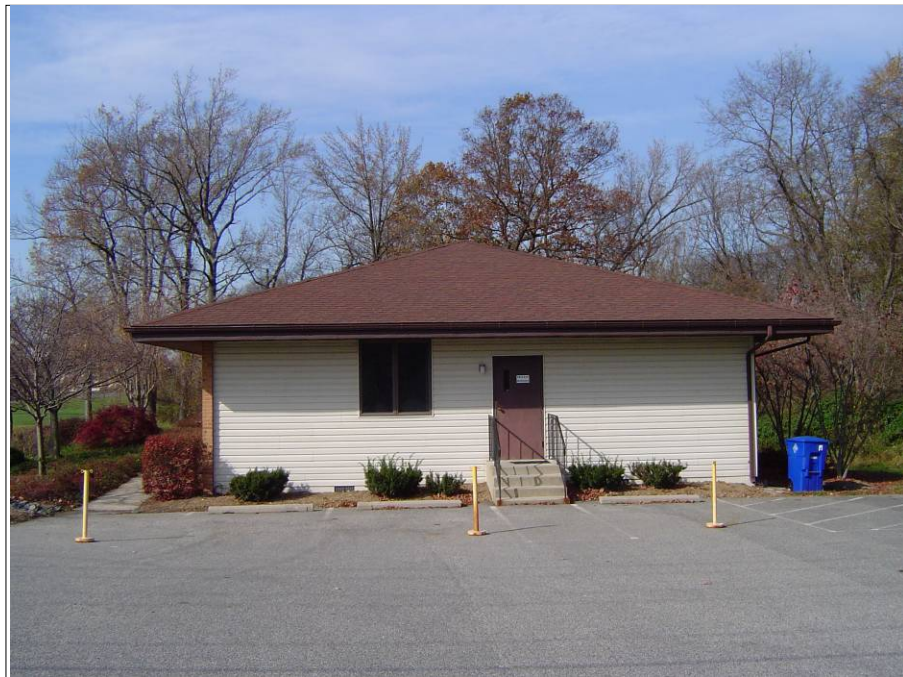
Figure 3-20. APG Building 2006: Side View of the East Exterior (to the right is N)
