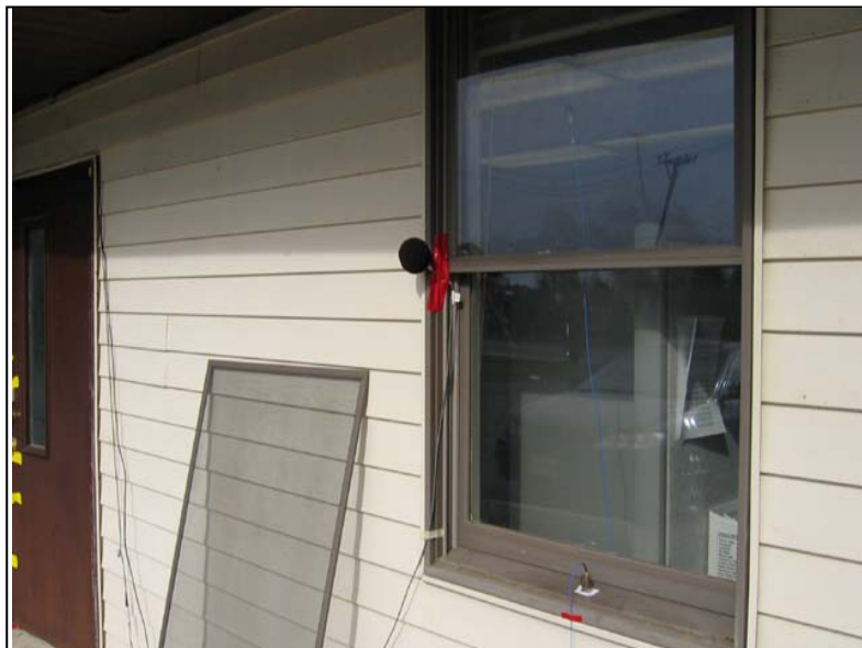
Figure 3-7. Transducers On and Around Window at APG Site C, Building 2001
