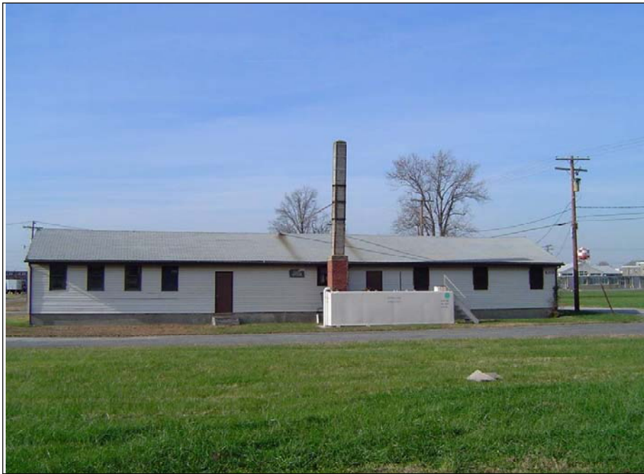
Figure 3-39. APG Building 4031: View of the North Exterior (to the right is W)
