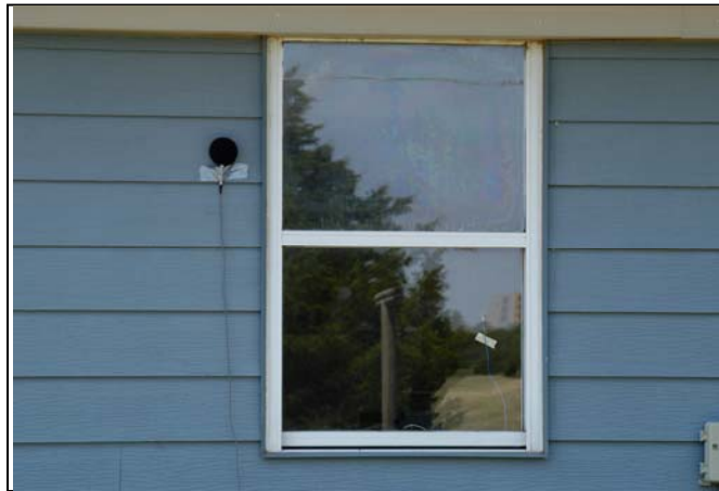
Figure 3-54. Accelerometer Placement On and Around Window, Building 6961B, Exterior
