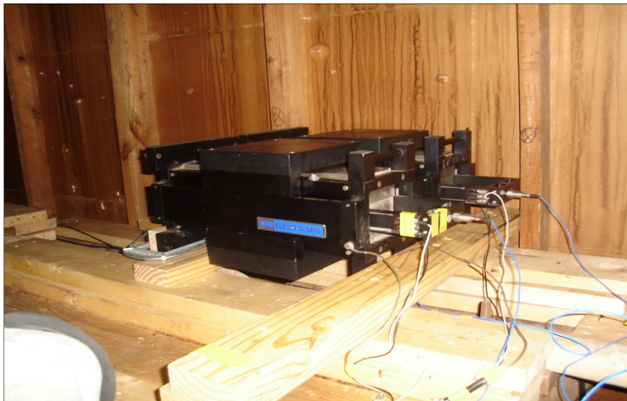
Figure 3-59. Shaker Installation at Building 216, Fort Sill
