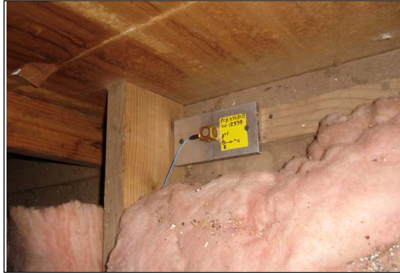
Figure 3-58. Transducer Installation at Building 216 Attic Level
