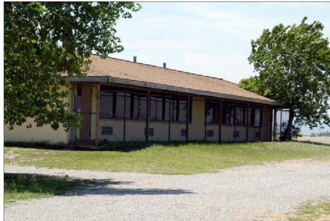
Figure 3-46. Building 6482 at 45W, Fort Sill
