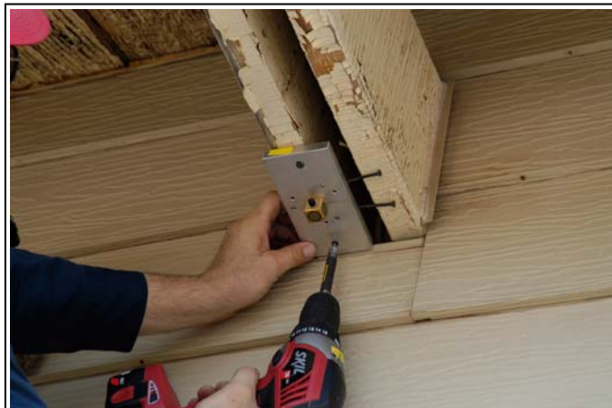
Figure 3-52. Installation of Triaxial Accelerometer, Building 216
