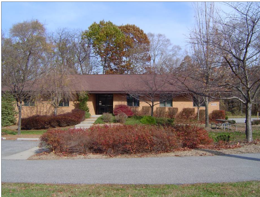
Figure 3-18. APG Building 2006: View of the Front (south) Exterior (to the right is E)
