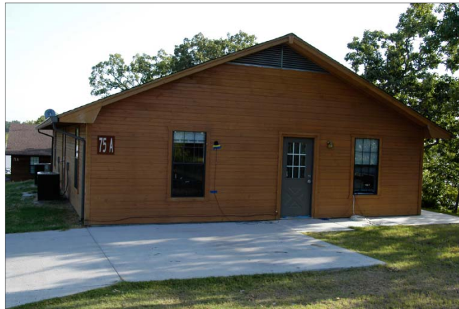
Figure 3-69. MCAAP Building 75A (Instrumented Window to Left)
