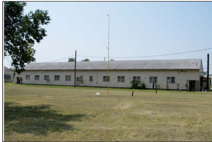
Figure 3-48. Building 216 (Warehouse) at Fort Sill ( Propagation Stack in Foreground )
