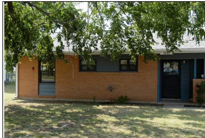
Figure 3-49. Building 1230, Fort Sill ( Instrumented Window on Left Side )
