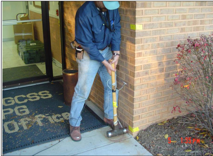
Figure 3-34. APG Building 2006: Close Up View of Front Door Entrance (to right is S) In this view the hammer has impacted the brick veneer wall near the bottom (Location J in Figure 3-32)
