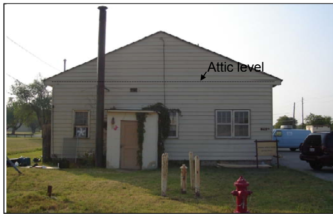
Figure 3-56. Elevation View of One End of Building 216, Warehouse
