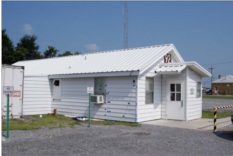
Figure 3-75. MCAAP Building 92: Instrumented Window and Top Corner Seen
