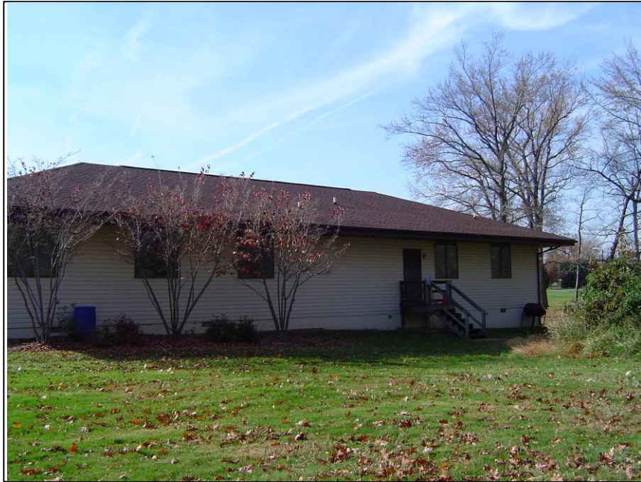
Figure 3-19. APG Building 2006: View of Back (north) Exterior (to the right is W)
