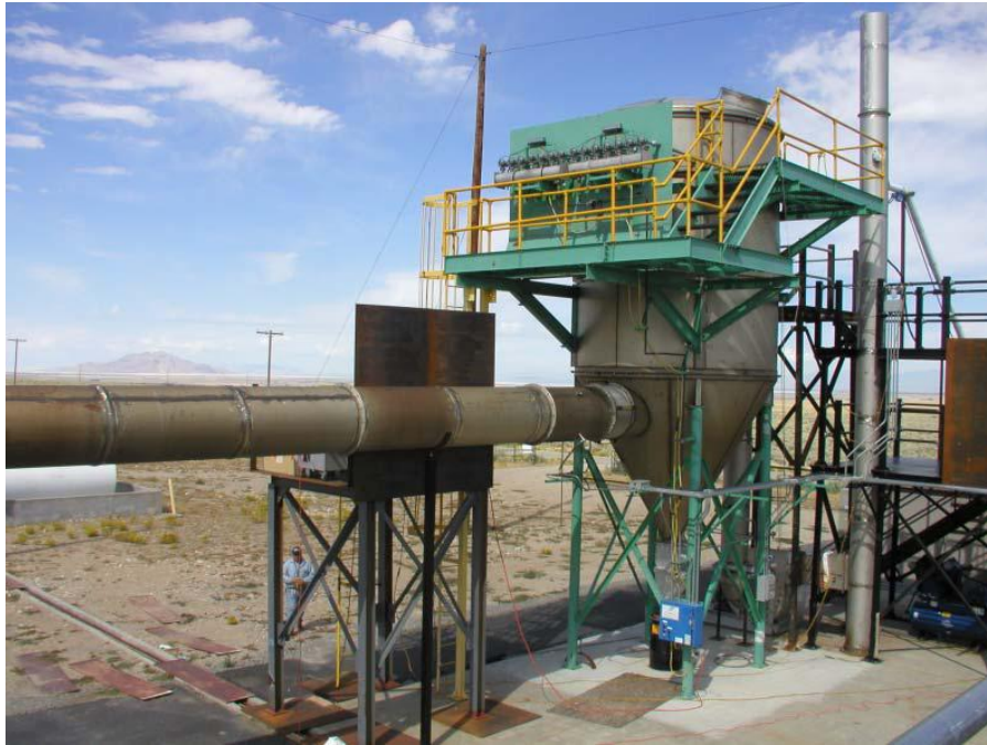
Figure 12. Sampling location for ABF-LIPS and reference method during September 2005 test on platform prior to baghouse. (platform is center left accessing horizontal duct)
