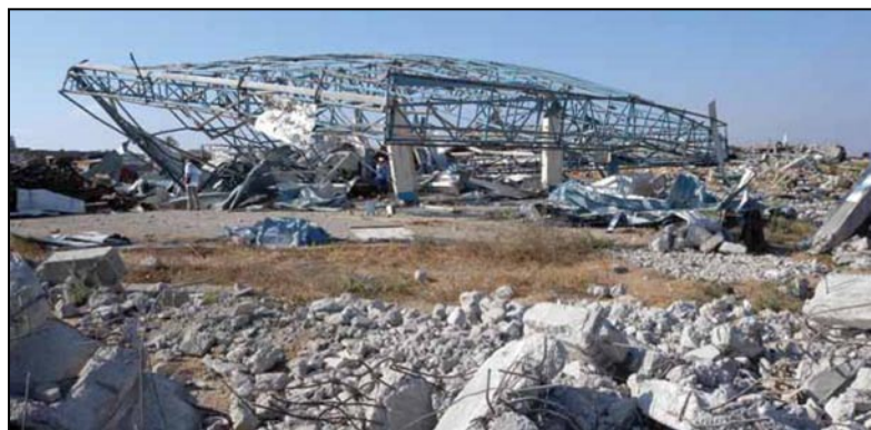
Figure 3-19: Destroyed Gas Station in Northern Gaza
