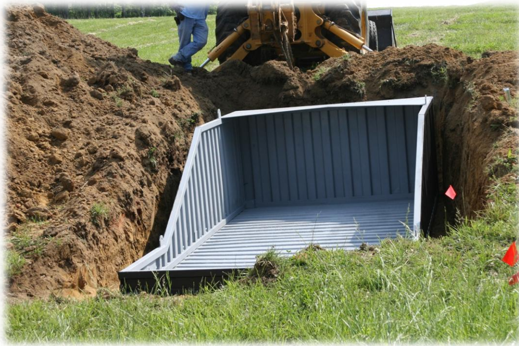
Figure 7. Fabricated connex unit after being lowered into the excavated berm.
