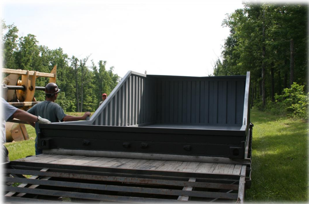
Figure 4. Painted containment berm prior to installation.
