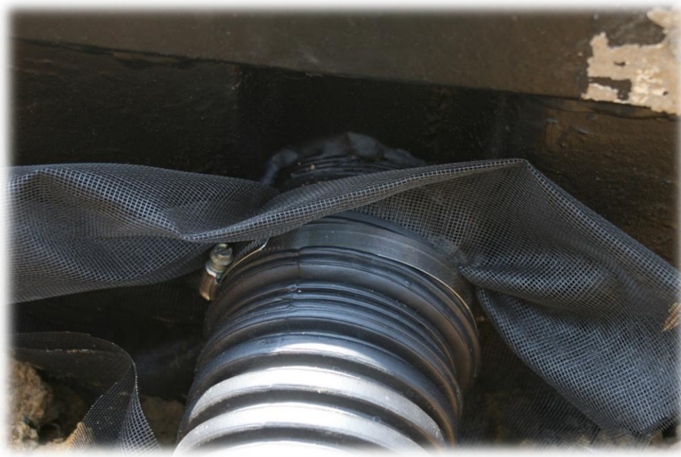
Figure 8. Placement of drainage port for the Containment Berm Unit.
