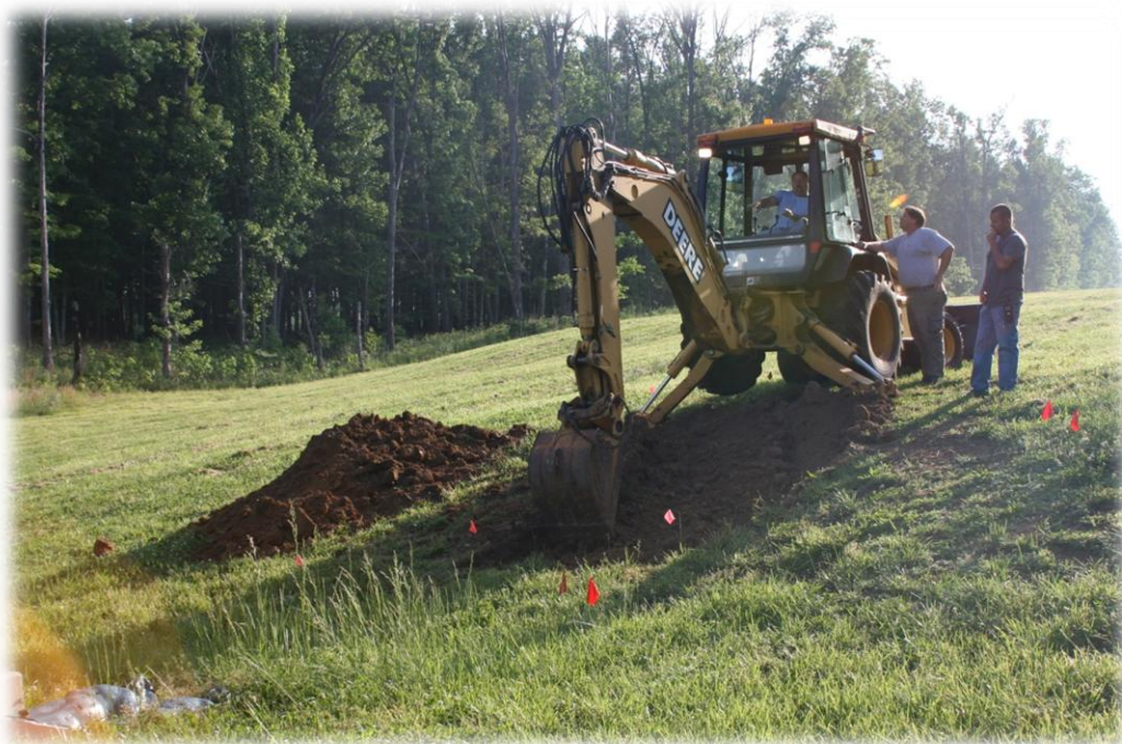
Figure 5. Initial excavation using a backhoe, showing marking flags.
