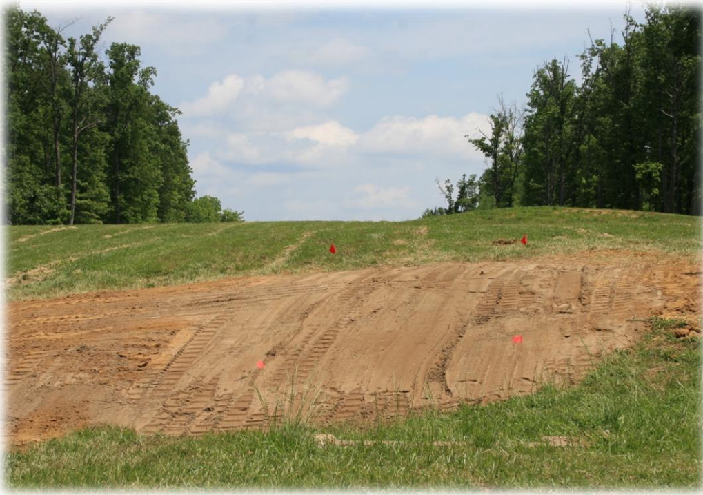
Figure 11. Completed Containment Berm Unit after re-grading.
