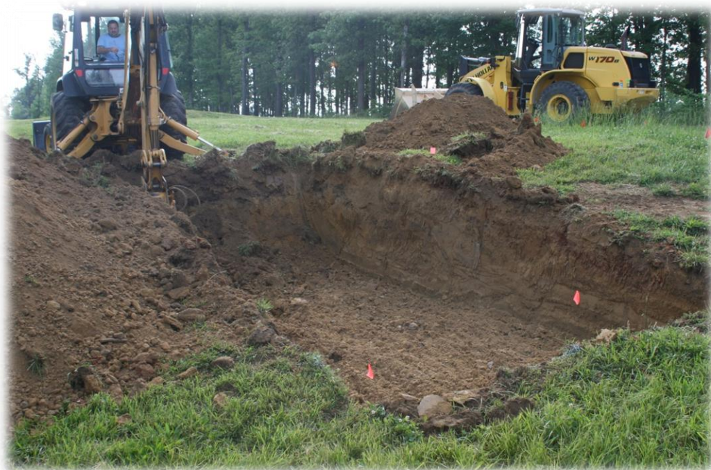
Figure 6. Final excavation at a depth ranging from 2 to 5 feet.
