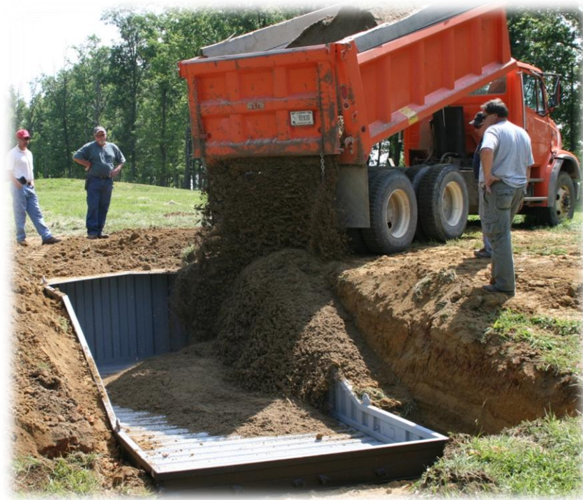
Figure 10. Filling Containment Berm Unit with sand and metal stabilizing soil amendment.
