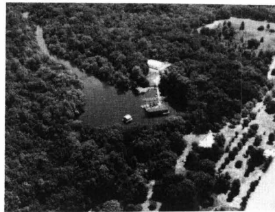
Leesburg Facility- Calibration Range (86)
