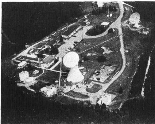
Waldorf Antenna Site
