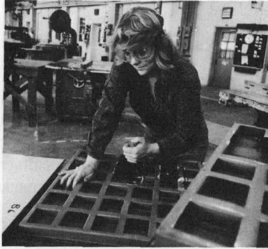
Modifying Computer Room Floor Tiles
