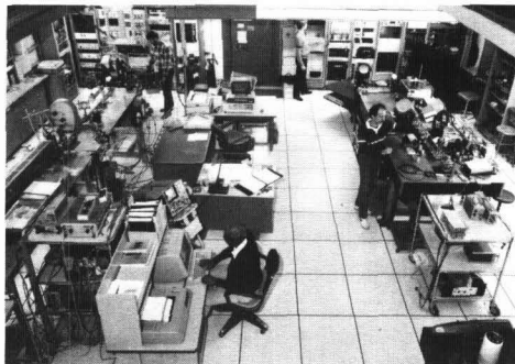
The Missile Seeker Evaluation Facility is a computerized facility that is used to evaluate optical countermeasures to infrared missile seekers and infrared imaging sensors.
