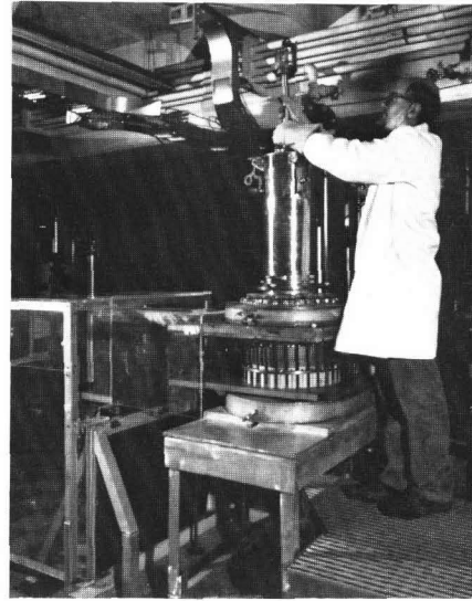
High-magnetic-field apparatus for spectroscopic characterization of materials
