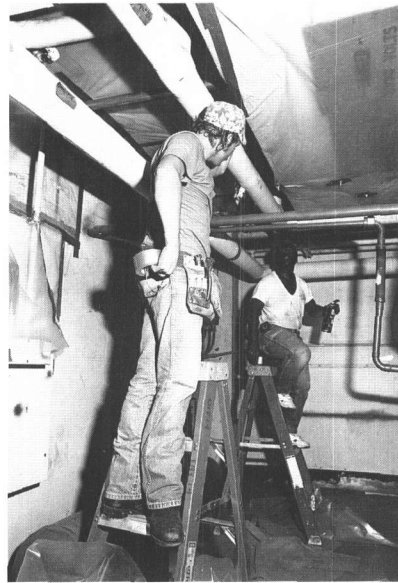
Asbestos removal work in progress
