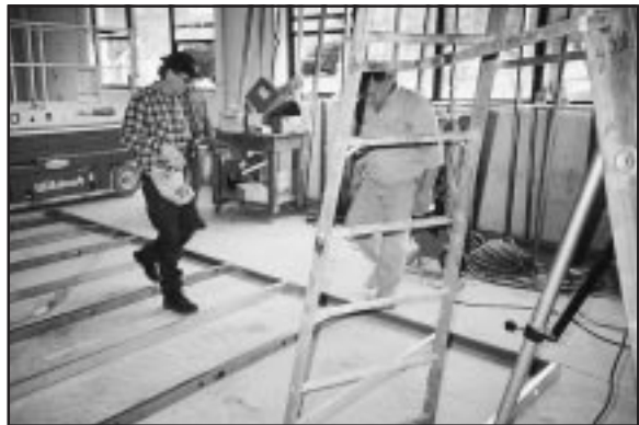
Renovation of Acoustics Division facility
