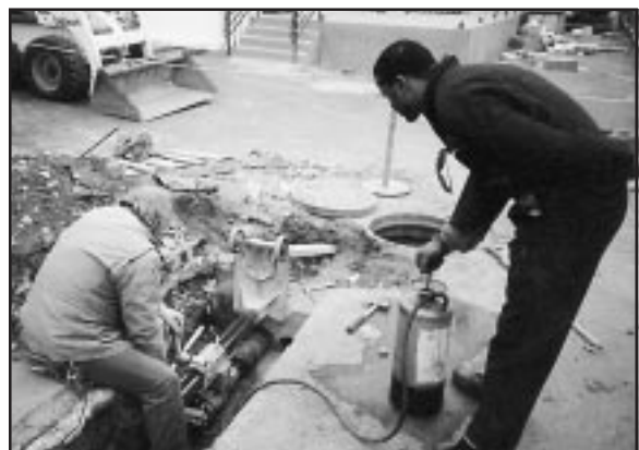
Installing new communication duct lines to service Information Technology Division's renovated Computational Science facility
