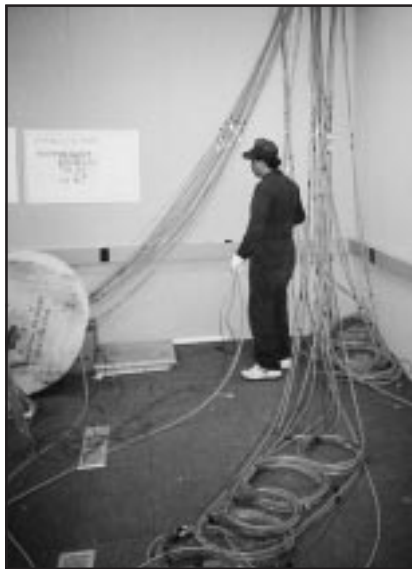
Installing fiber optic lines
