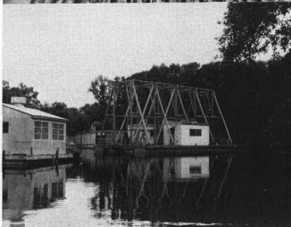
LEESBURG FACILITY- CALIBRATION BARGE
