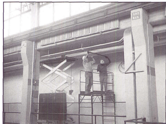
Mezzanine of Remote Sensing Division under construction
