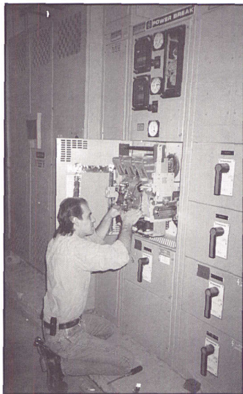
Main switch gear undergoing emergency repair
