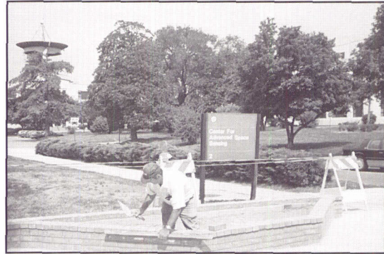
Entrance to Remote Sensing Division under construction
