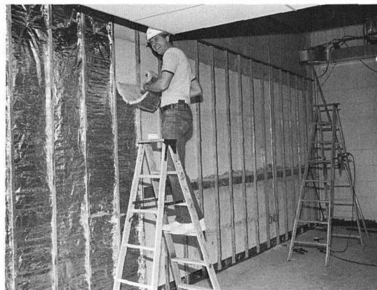
Electronics laboratory under construction
