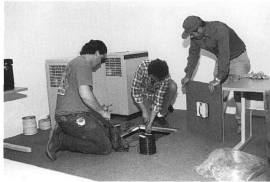
Computer room installation
