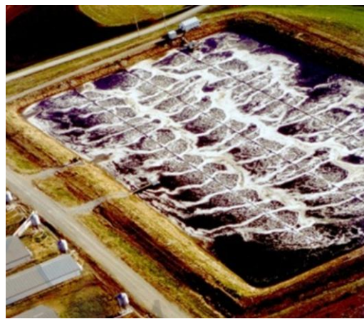
Figure 4. Mechanically Aerated Lagoon (Photo: Wikipedia Commons)
