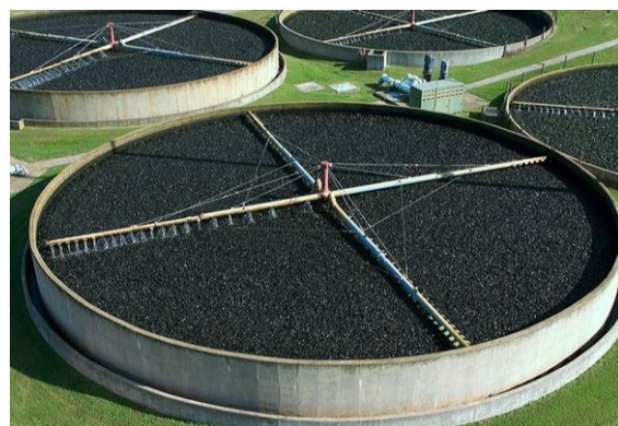
Figure 5. Trickling Filter (Photo: Brian Hayes, “Infrastructure: A Field Guide to the Industrial Landscape”)
