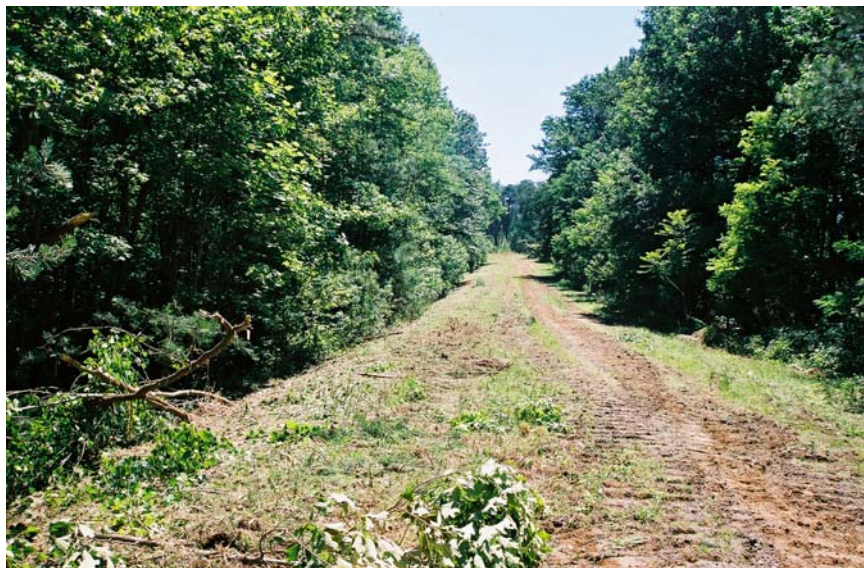
Figure 15 Downhill Embankment, After Shredding
