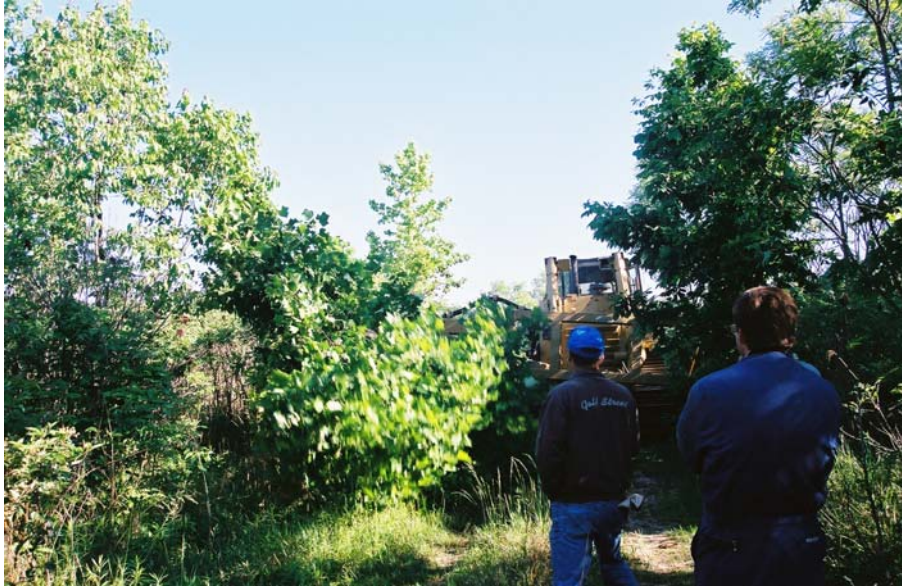
Figure 10 Bringing Down 10 m Tree
