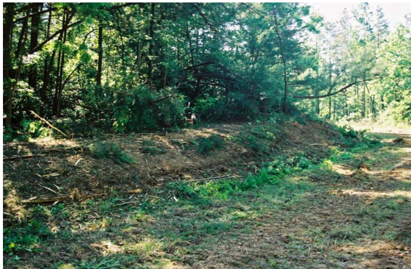
Figure 13 Uphill Embankment, After Shredding
