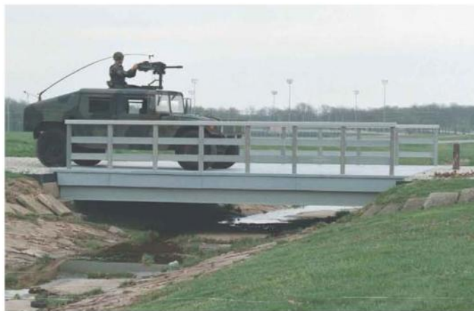
Figure 1. Thermoplastic composite lumber bridge at Fort Leonard Wood, MO.
