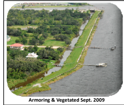
Figure 33. ARVS behind existing I-wall.
