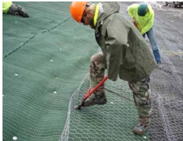
Figure 38. Connection of ARVS to mattress.
