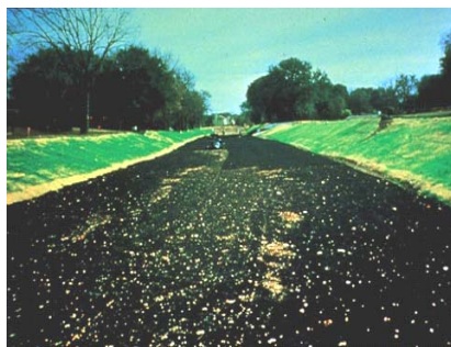
Figure 19. TRM channel application.
