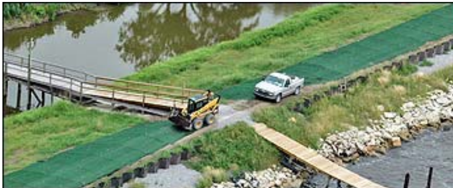
Figure 7. Levee project – construction traffic on permanent vegetated armoring system.
