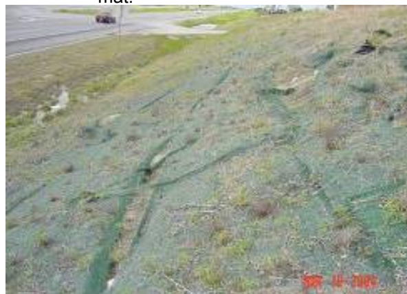
Figure 3. Insufficient tensile strength and poor seams can lead to mower damage.
