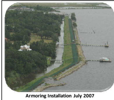
Figure 32. ARVS on earthen levee.
