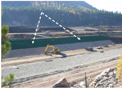
Figure 37. ARVS with 9-in. Reno mattress.
