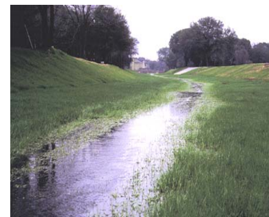
Figure 21. Fully vegetated TRM.
