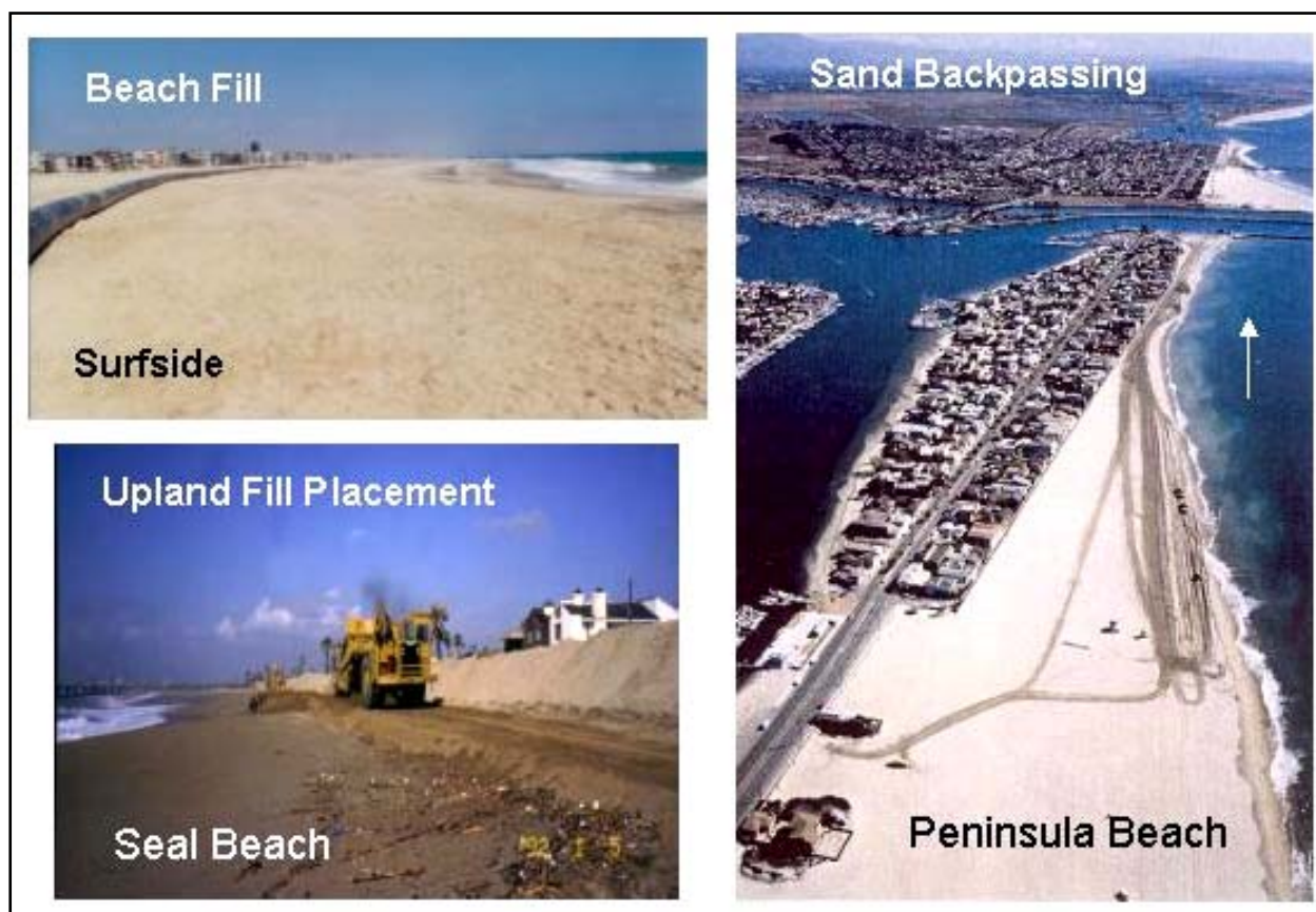
Figure 22. Photographs of mitigation for the three hot spots along southern California coast showing pipeline fill renourishment from offshore borrow area at surfside, upland fill placement at Seal Beach and truck haul backpassing at Peninsula Beach (courtesy of Chuck Mesa, Los Angeles District)
