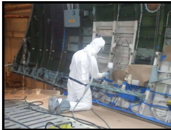
Figure 2: Chine coves being painted
