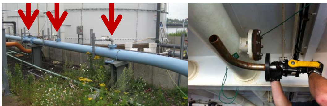
Figure 11. The three sample ports used for biological sampling at the Great Ships Initiative (left image) and one sample port used at the Golden Bear Facility (right image). The red arrows identify the sample ports in the left image.
