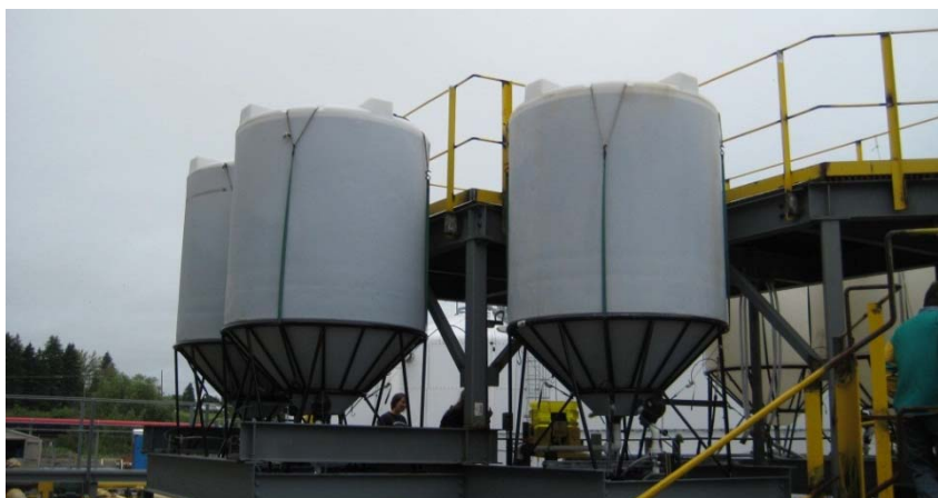
Figure 9. Biological sample collection tubs at the Great Ships Initiative; tubs are white with conical bottoms.
