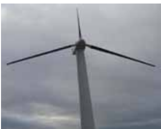
DoD IG reviewed energy conservation wind turbine projects.
