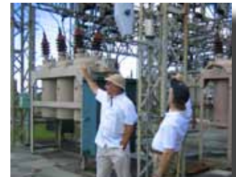
DoD IG assessed the infrastructure requirements for Guam.
