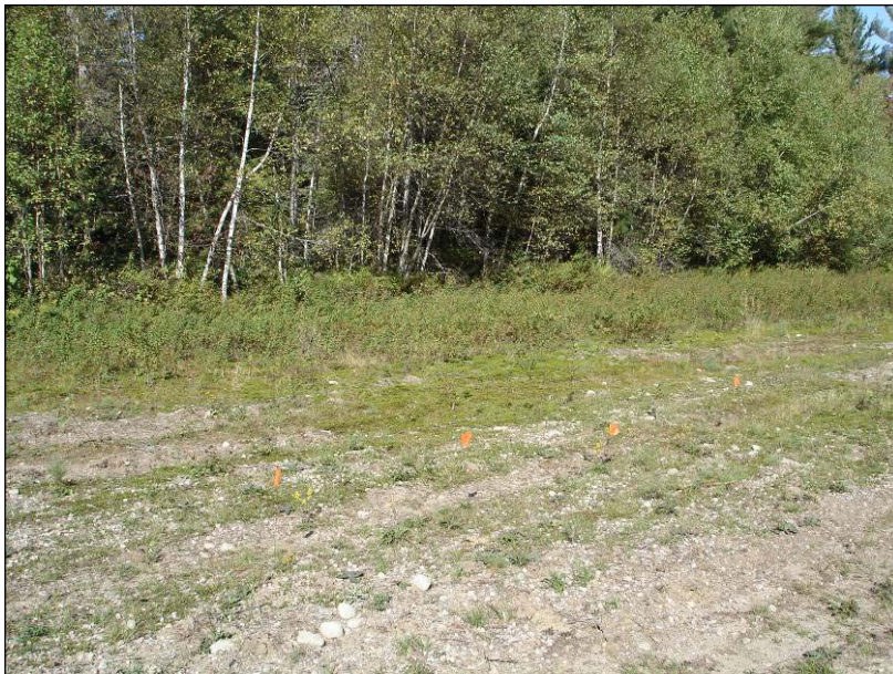
a) Before installation of the propellant lines.
