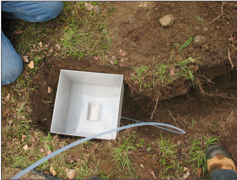
Figure 5-11. Installation of lysimeters at Carpiquet.
