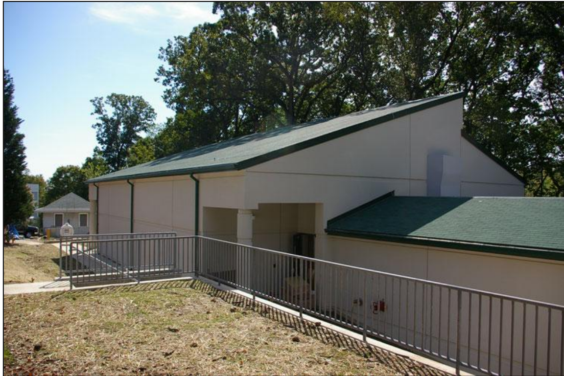
Figure 11. New clock building.
