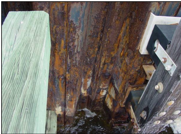
Figure 9. Typical corrosion on Pensacola steel sheet pile before surface preparation.
