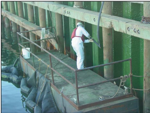
Figure 19. Coating application on Pensacola SSP.
