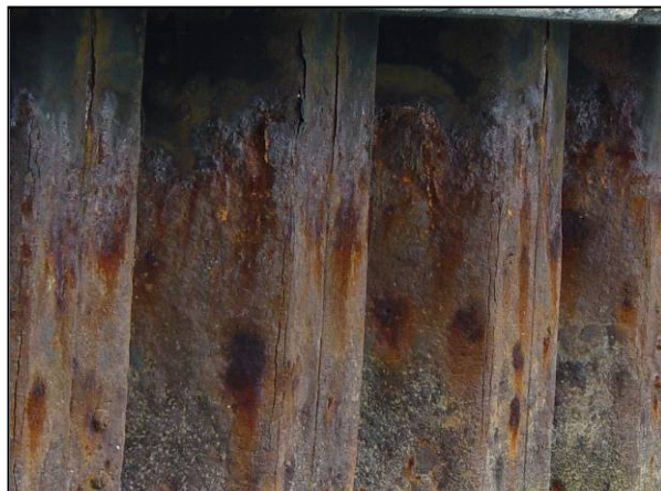
Figure 11. Typical corrosion on San Diego steel sheet pile before surface preparation.
