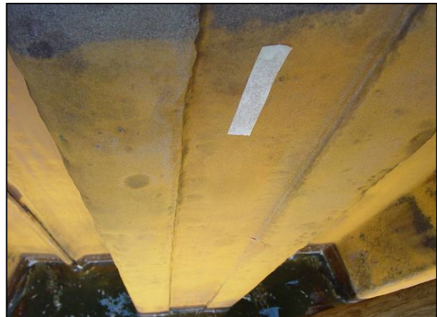
Figure 16. Pensacola SSP after flash rusting and before coating application.
