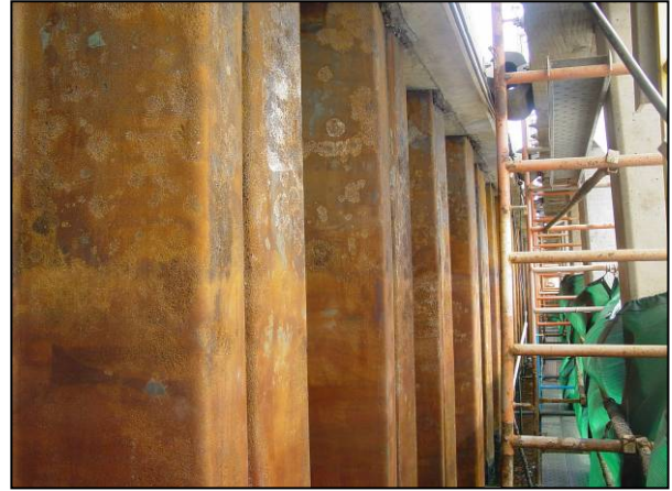
Figure 18. San Diego SSP after flash rusting and before coating applications.
