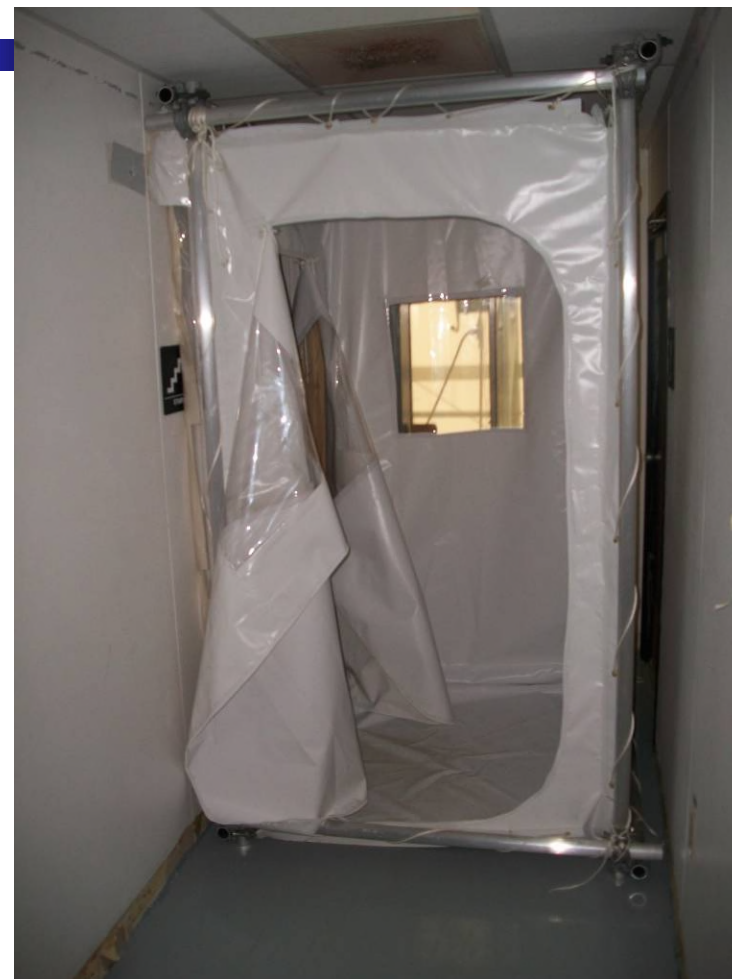
PBF-632 Airlock between 2 nd and 1 st floor low and high simulant concentration areas (required for cross contamination control)
