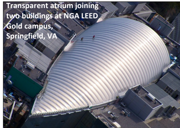
Photo: U.S. Army Corps of Engineers
